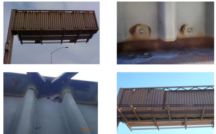
Image 1: Typical corrosion damage of in-service box
