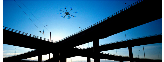
Picture 1: Unmanned aerial vehicle inspecting infrastructure
