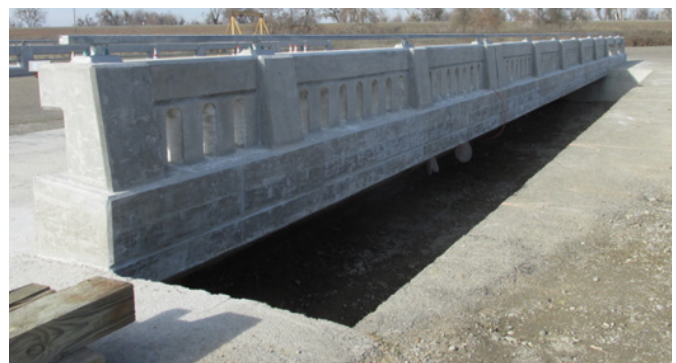
Image 3: Type 86H Concrete Barrier looking North West
