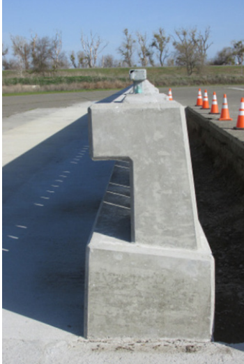
Image 4: Type 86H Concrete Barrier looking North
