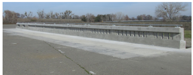
Image 2: Type 86H Concrete Barrier looking North East
