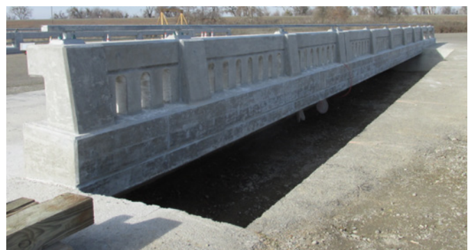
Image 3: Type 86H Concrete Barrier looking North West
