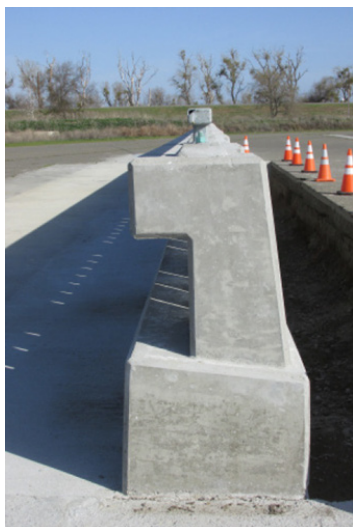
Image 4: Type 86H Concrete Barrier looking North
