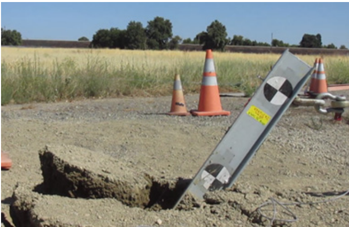
Image 2: Static Test of New Compaction Method 2.
