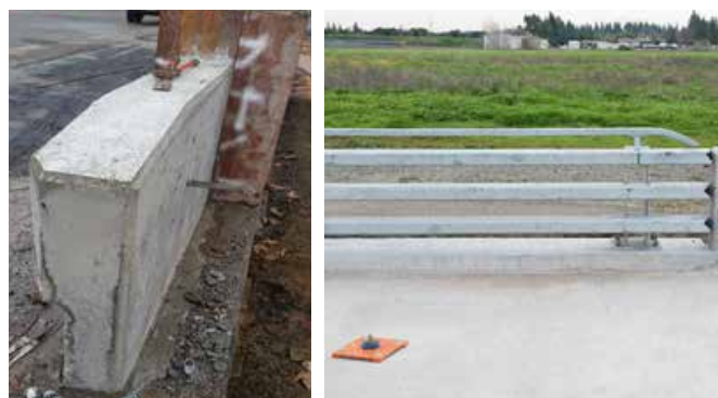
Picture 3: Caltrans Standardized Buttress
