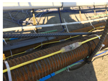
Image 4: TIP wires for thermal measurement
