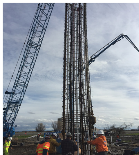
Image 5: Drilled shaft construction
