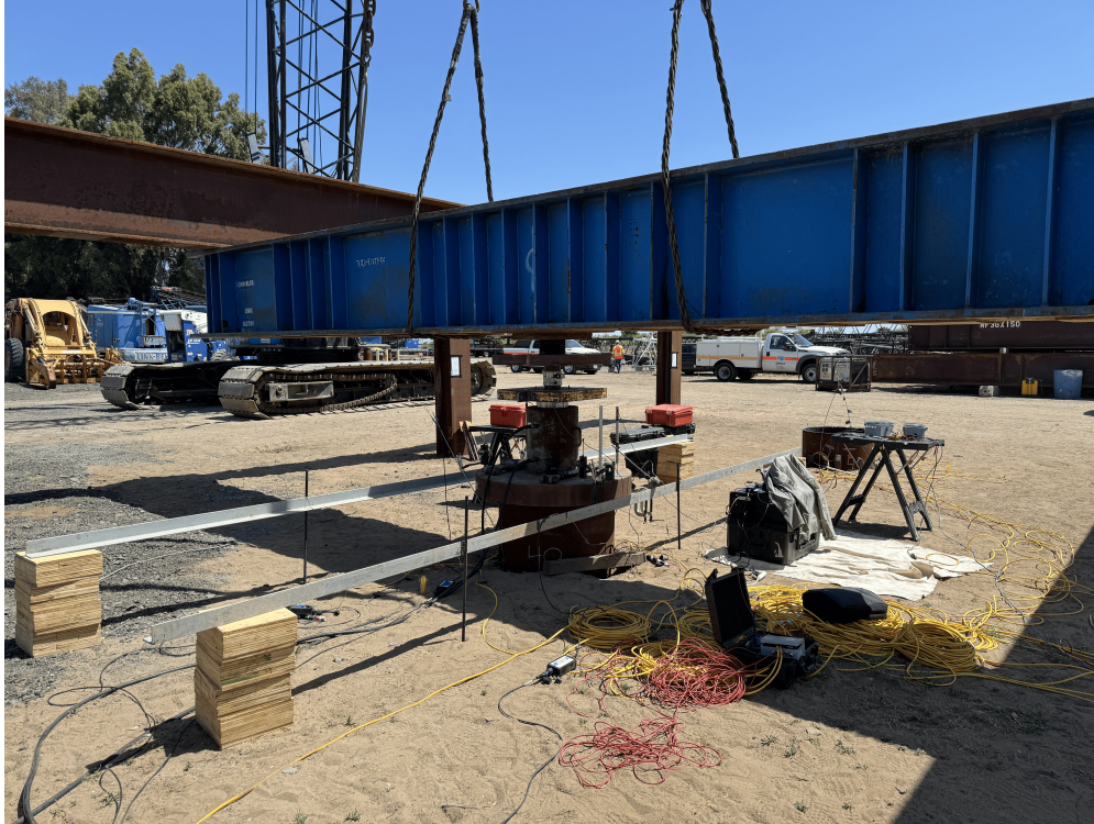
Figure 13: Example of pile load test configuration during testing.
