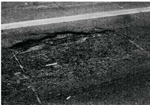
Pavement failure near installation
