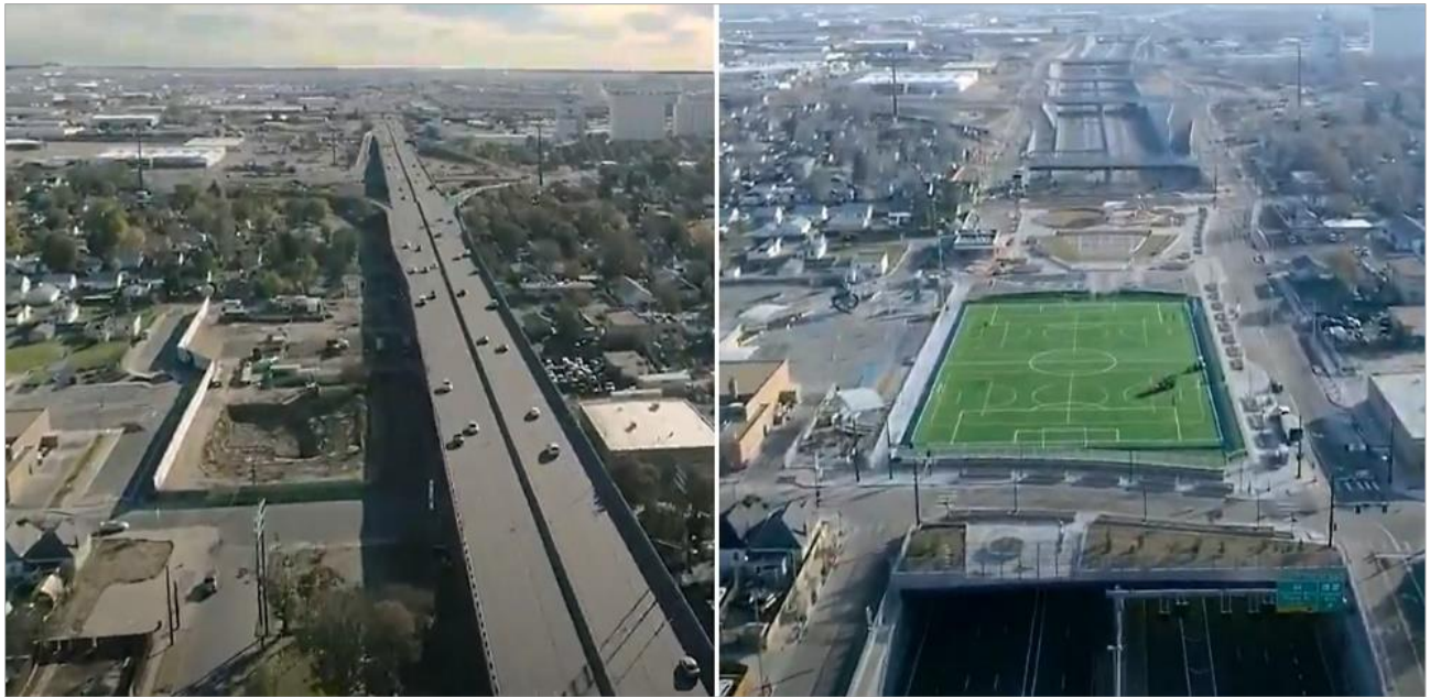
Figure 7. Aging viaduct removed in the Central 70 project (left); 4-acre cover park over the lowered interstate (right) (Source: Innovator Newsletter .)
