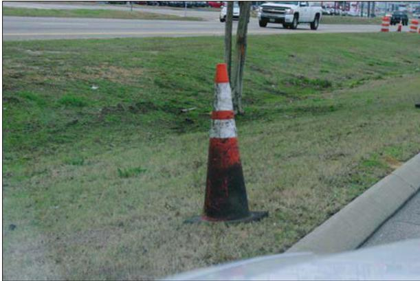
**X** Sprayed with Asphalt
