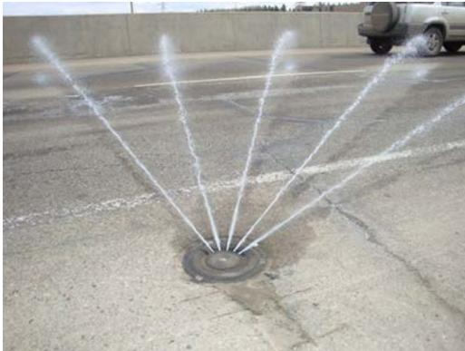
Figure 6. Bridge Deck Integrated Brine Spray
