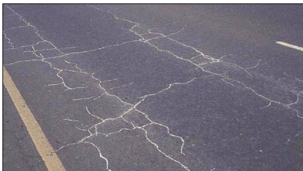
Figure 3.4: Block cracking on an FDR-C pavement (note pumping of fines through cracks).
