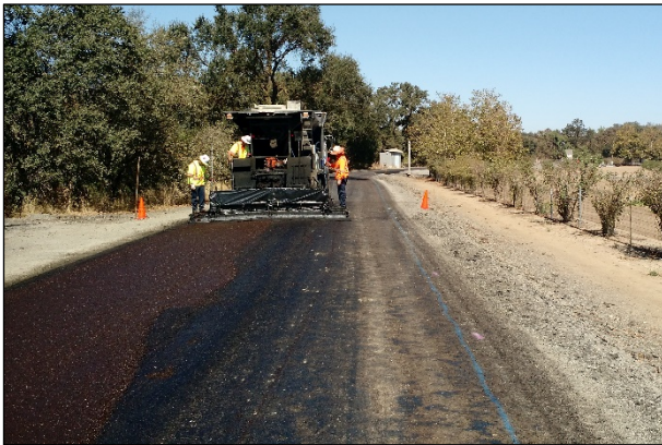
Figure 5.37: First microsurfacing pass.
