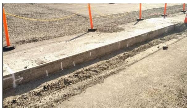
Figure 2.28: Wet FDR-C test section.
