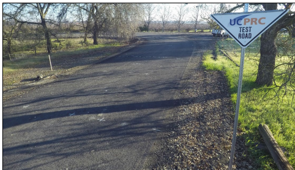
Figure 6.1: FDR-C Test Road.
