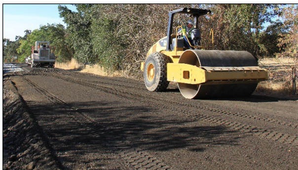
Figure 5.10: Final compaction with a smooth drum roller.
