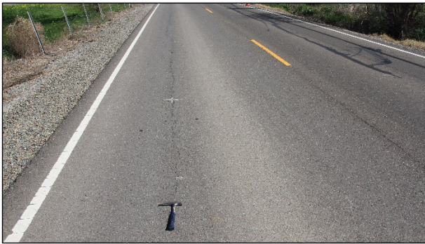
Figure 2.1: CR32B: Example longitudinal cracks.
