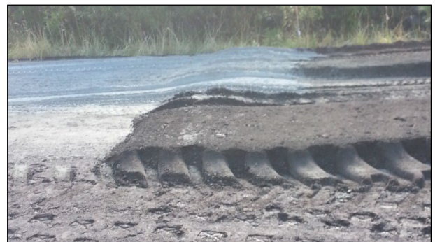
Figure 2.13: Cement spreading overlaps.
