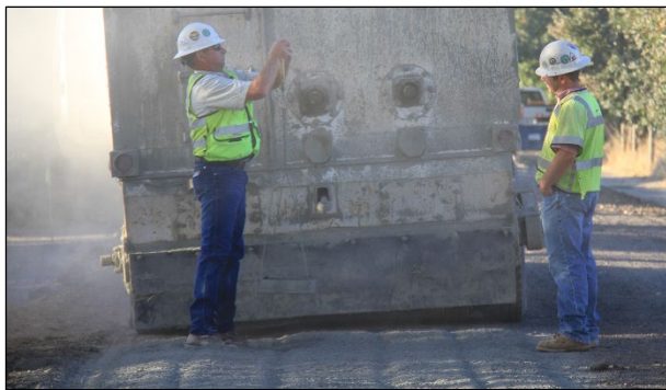
Figure 5.4: Checking cement spread rate.
