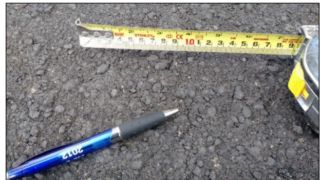
Figure 6.2: Narrow crack width of drying shrinkage crack at first appearance.
