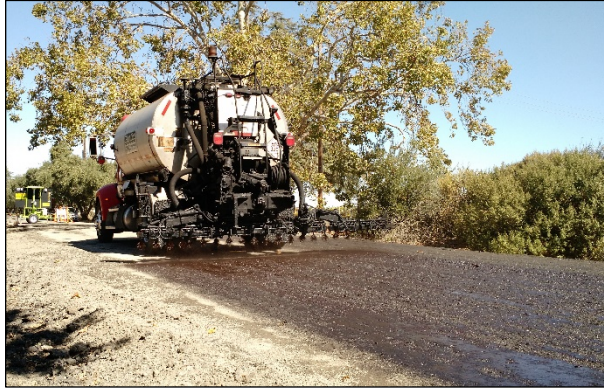
Figure 5.36: Prime coat application.
