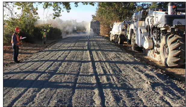
Figure 5.5: Checking cement spread overlaps.
