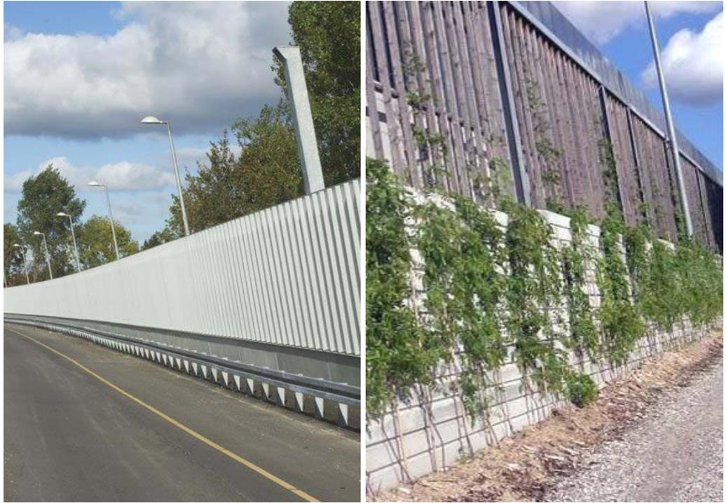
*Figure 5.4. Close up of the noise barriers designed for the M3 project (roadside left and urban side right).*
