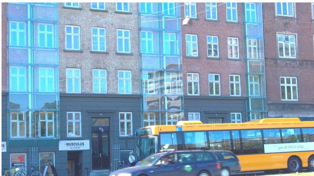
*Figure 6.8. Glass covering has been mounted as noise insulation for bedrooms and living rooms at the façade of a multi-storey apartment building along a highway in Copenhagen, Denmark. Cleaner air from the backside of the building is used for ventilation between the glass covering and the existing windows. The noise abatement was financed as a part of an overall renewal of the building.*
