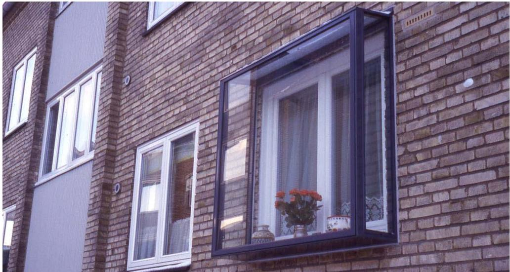
Figure 1.1. Façade insulation by applying a “glass box” in front of an existing window of bedroom or living room. Example from an apartment building in Århus, Denmark [10].
