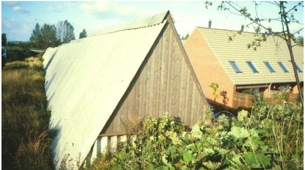
*Figure 7.2. A new district of row houses constructed along an existing highway. A common carport facility was constructed as a two storey high noise barrier.*
