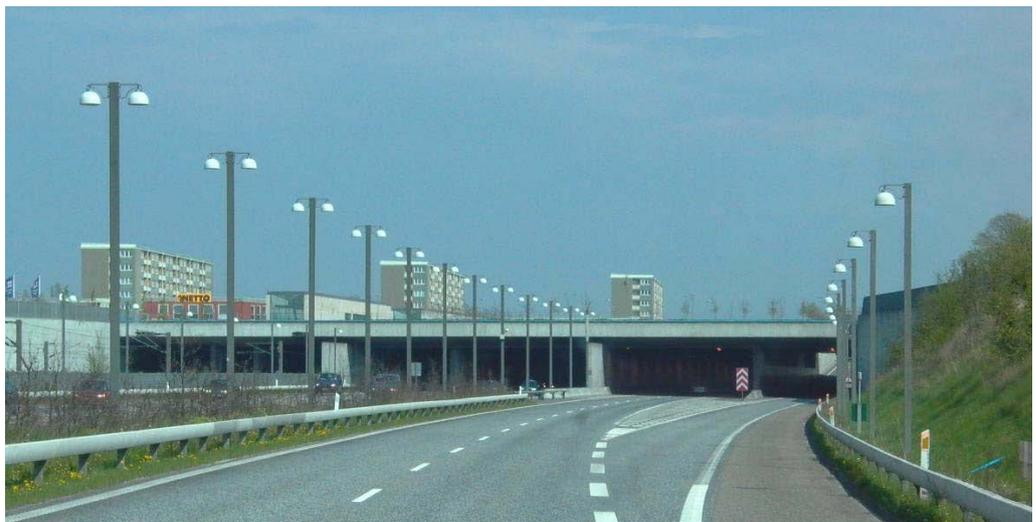
Figure 4.5. 700 m long section of the new highway to Copenhagen airport, Denmark was constructed as a cut and cover strategy in order to reduce the noise exposure for some nearby multi-storey apartment buildings.
