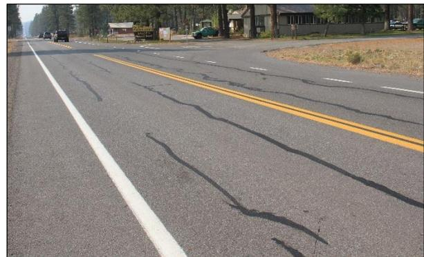
**Figure 3.6: Alligator-A cracking on a PDR project.**
