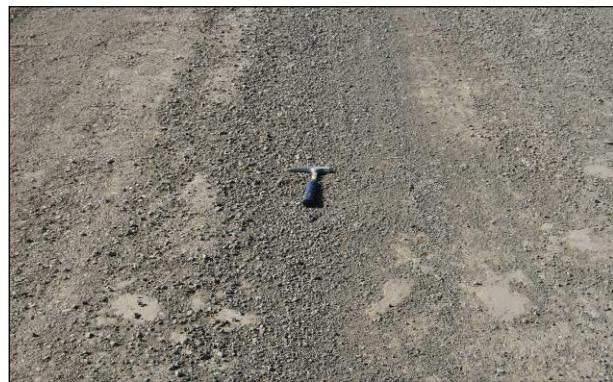
**Figure 6.122: Unacceptable surface prior to tack coat application.**
