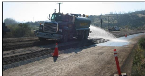
**Figure 6.76: Separate water application behind recycler (FDR).**
