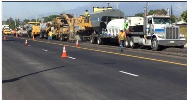
Figure 1.4: Partial-depth recycling train (multi-unit).
