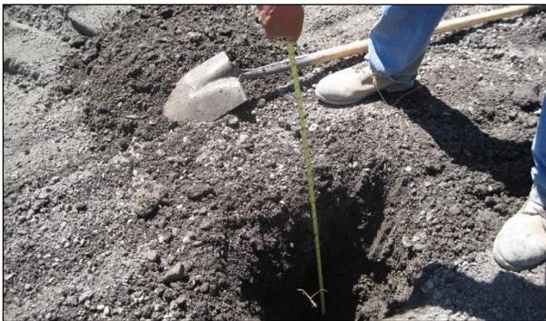
Figure 6.46: Checking recycling depth on an FDR-C project.
