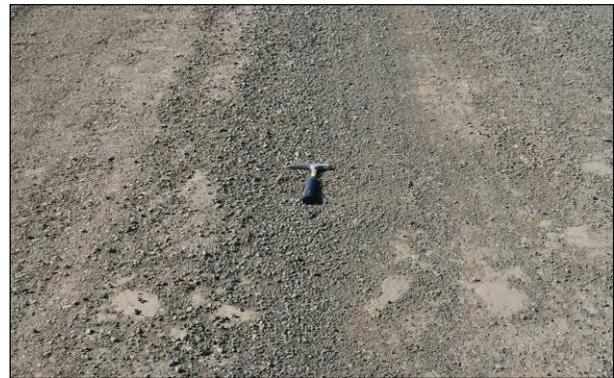
**Figure 6.122: Unacceptable surface prior to tack coat application.**
