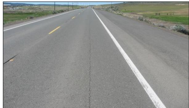
**Figure 6.72: Reflected longitudinal crack in area of cement spread overlap (FDR-C).**
