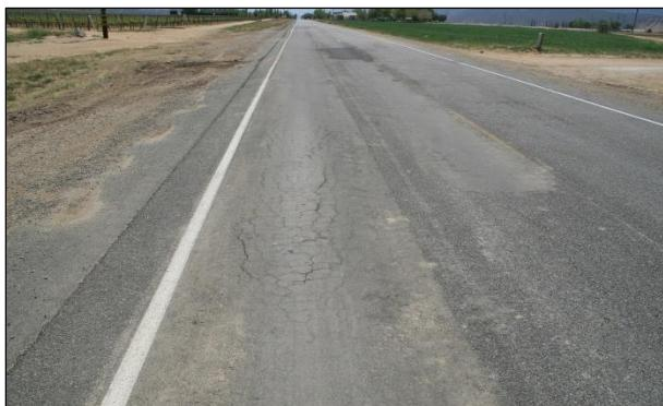
**Figure 2.31: Early failure in wheelpath repairs.**
