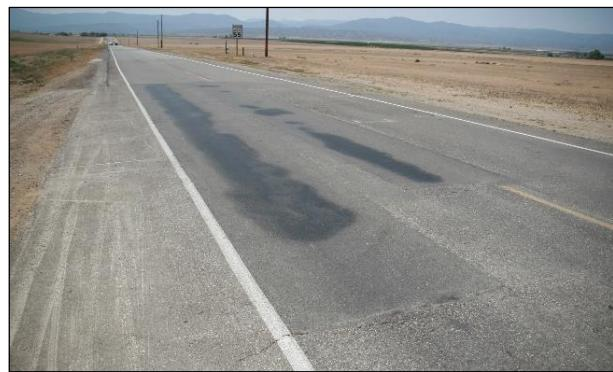
**Figure 2.32: Bleeding in wheelpath repairs.**
