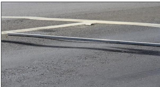
**Figure 2.13: Example top-down distresses: Surface ruts/densification.**
