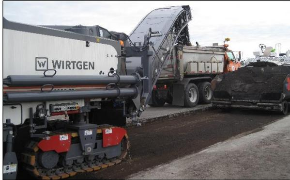
**Figure 6.81: Removing excess material on a PDR project.**
