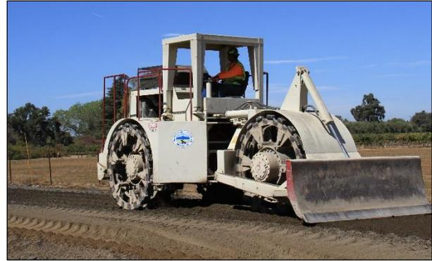
**Figure 6.16: Segmented padfoot roller on an FDR-C layer.**
