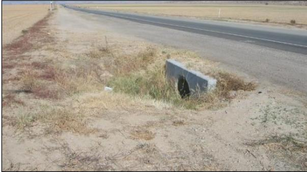
**Figure 2.33: Blocked side drain and culvert.**
