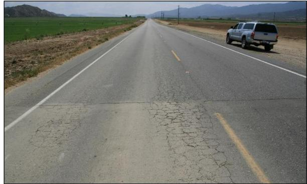
**Figure 2.3: Example early full-width patch failure.**
