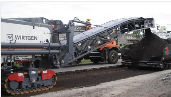
**Figure 6.79: PDR project with belt feed into paver.**
