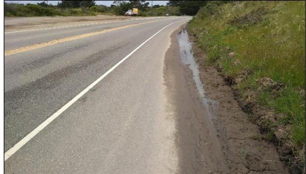
**Figure 2.7: Example drainage problem in cut.**
