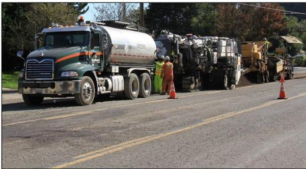
**Figure 6.6: Single-unit PDR recycling train.**
