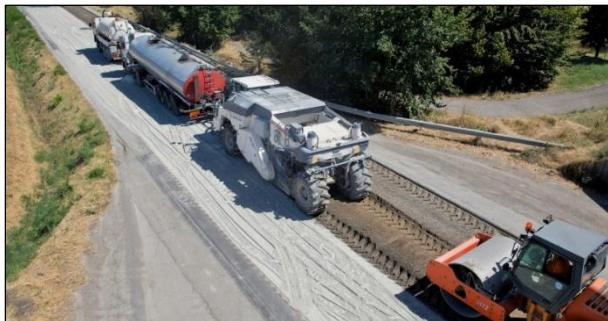
**Figure 6.8: Wheel-driven FDR recycling train.**
