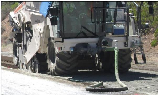
**Figure 6.21: Water leak during tanker change (FDR).**
