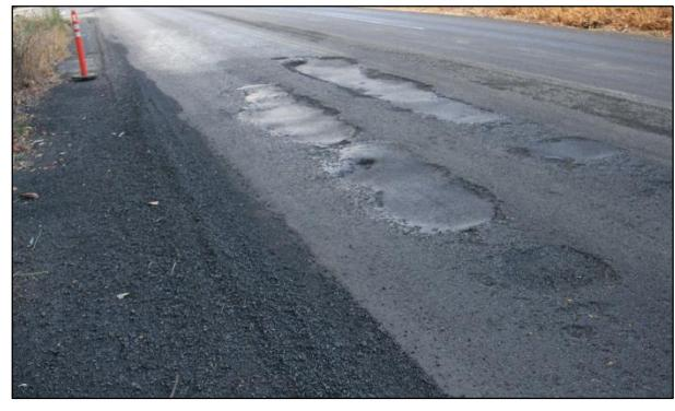
**Figure 6.52: Trafficked recycled layer with severe raveling (patched) (PDR).**
