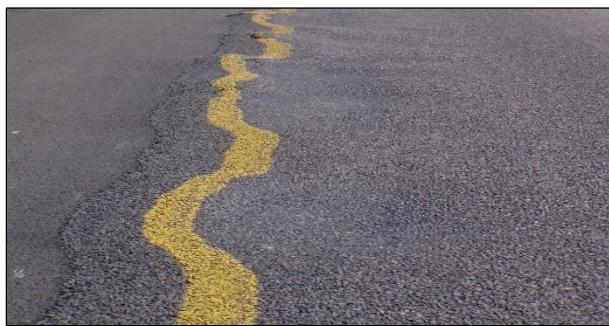
**Figure 2.15: Example top-down distresses: Mix
