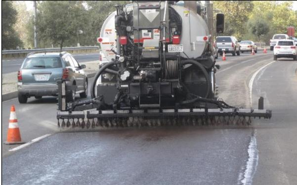
**Figure 6.108: Curing seal application on a PDR project.**
