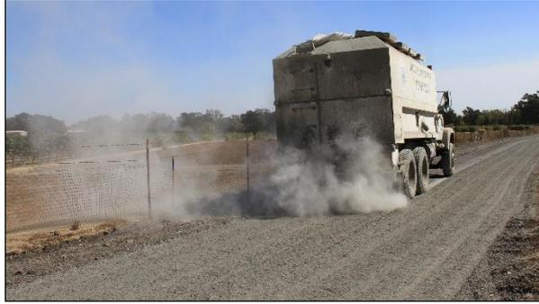
**Figure 6.12: Active filler/stabilizer spreader.**
