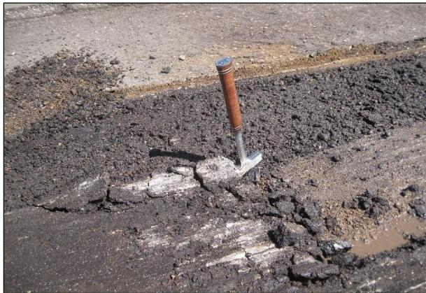
**Figure 6.53:** Thin, debonded layer on a PDR project.
