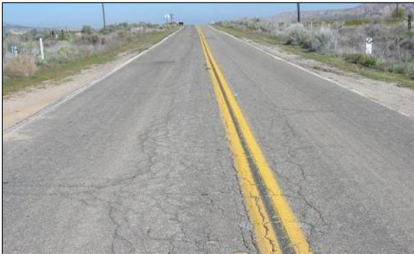
**Figure 2.4: Example alligator-B cracking.**
