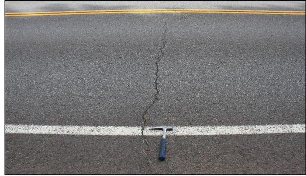
**Figure 6.20: Early shrinkage cracks in area of accumulated cement (FDR-C).**
