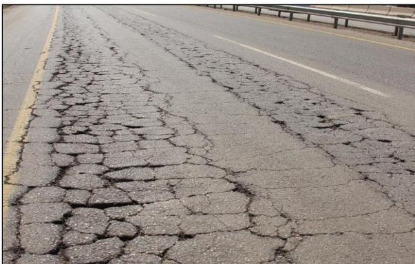
**Figure 2.27: Loose blocks in severe alligator-B cracking.**
