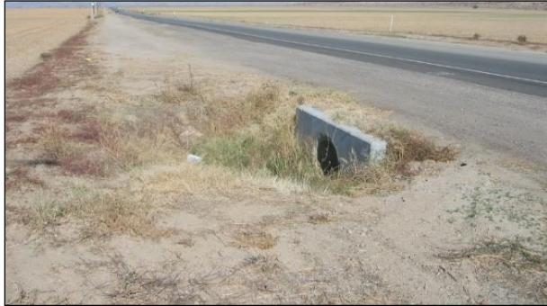
**Figure 2.33: Blocked side drain and culvert.**
