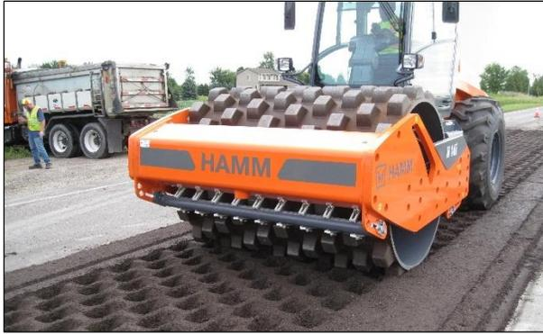
**Figure 6.15: Vibratory padfoot roller on an FDR-FA layer.**
