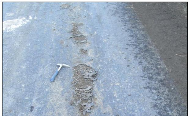
**Figure 6.118: Delaminated area exposed during shrinkage crack mitigation (FDR-C).**
