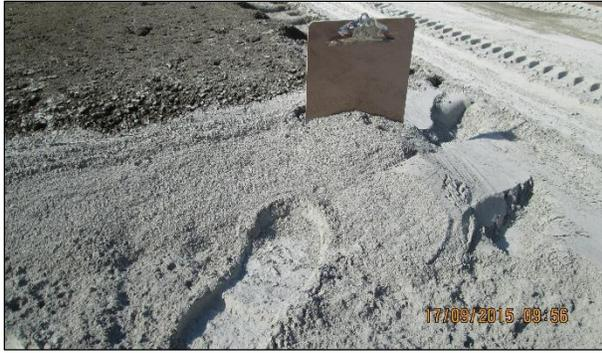
**Figure 6.19: Accumulated cement dragged by hose at end of recycling run (FDR-C).**
