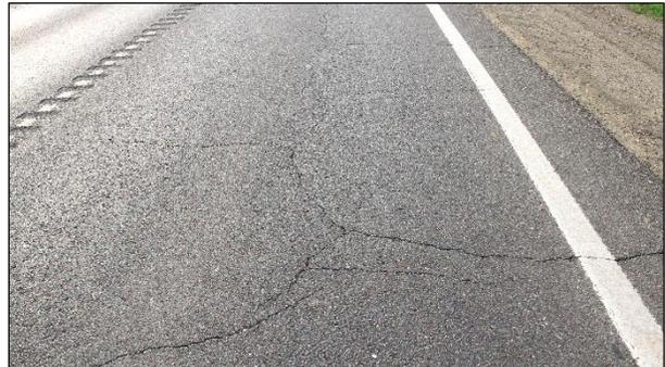
**Figure 2.20: Example bottom-up distresses: Block
