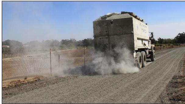
Figure 6.12: Active filler/stabilizer spreader.
