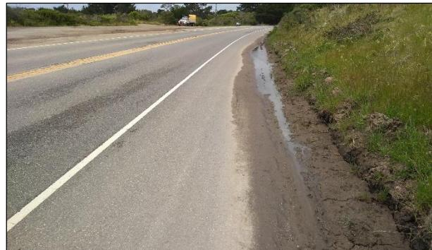
**Figure 2.7: Example drainage problem in cut.**
