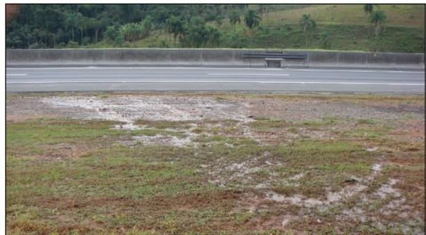
**Figure 2.38: Water flowing downslope into the road.**
