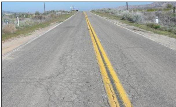
**Figure 2.4: Example alligator-B cracking.**
