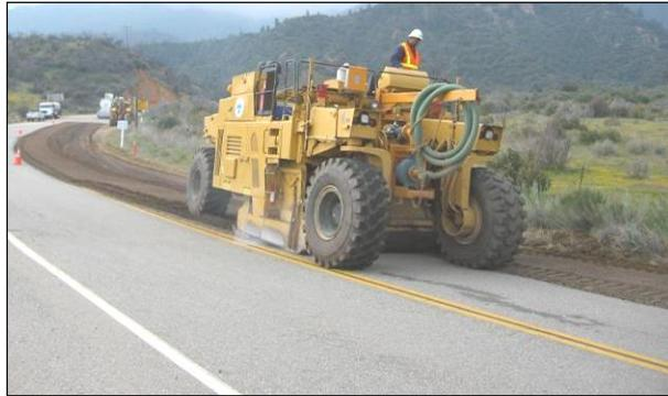
**Figure 6.55: Prepulverization on an FDR project.**
