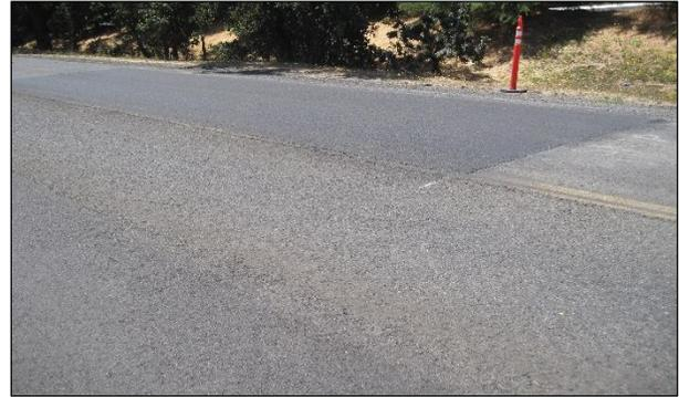
**Figure 6.120: Patched distressed areas prior to surfacing.**
