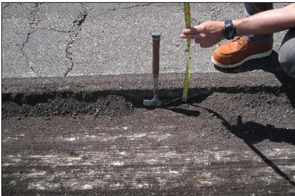
**Figure 6.27: Checking recycling depth on a PDR project.**
