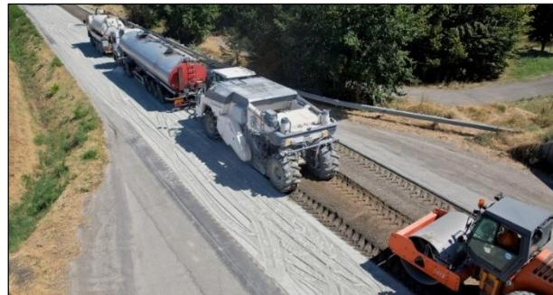
Figure 1.5: Full-depth recycling train (wheel).
