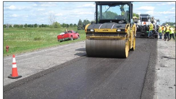
**Figure 6.84: Primary compaction starting with smooth-drum roller on a PDR project.**
