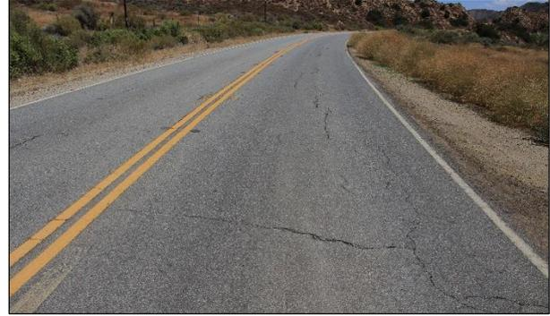
**Figure 6.78: Early cracking caused by poor moisture distribution in recycled layer (FDR).**
