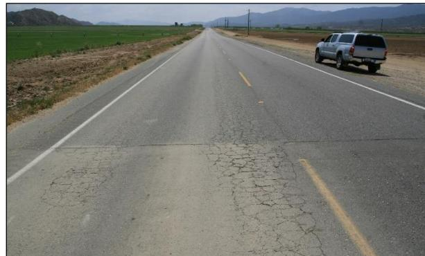
**Figure 2.3: Example early full-width patch failure.**
