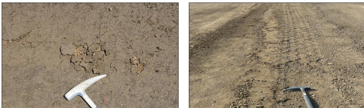
**Figure 6.102: Delamination after blading thin lifts of material during grading (FDR).**
