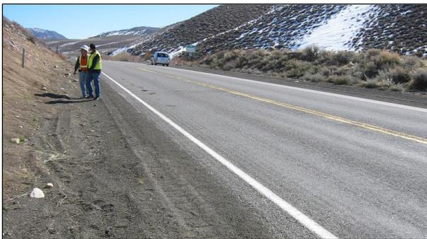
**Figure 2.37: Absence of drains below cut slopes.**
