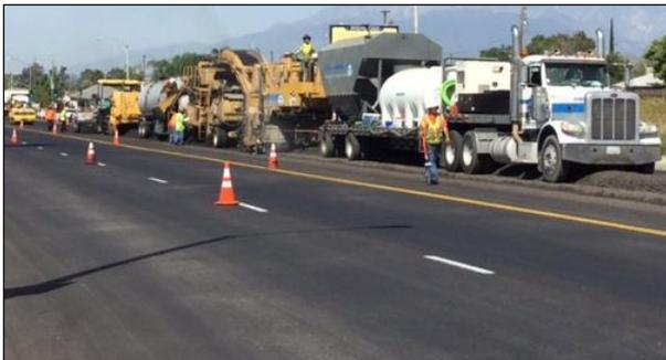
Figure 1.4: Partial-depth recycling train (multi-unit).
