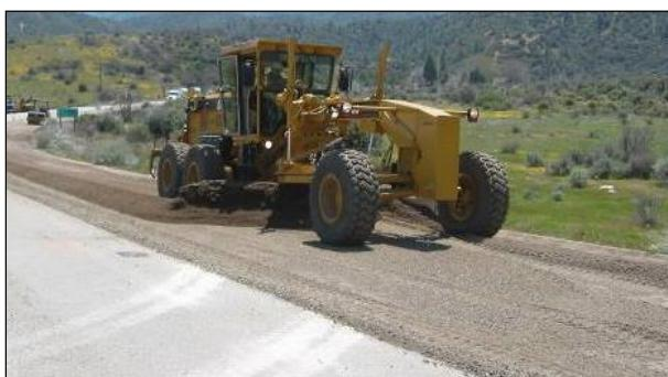
**Figure 6.99: Shaping and final leveling with a grader on FDR projects.**
