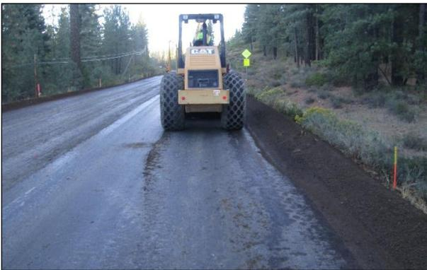
**Figure 6.117: Damage to emulsion curing seal during shrinkage crack mitigation (FDR-C).**
