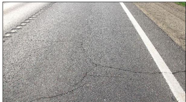
**Figure 2.20: Example bottom-up distresses: Block
