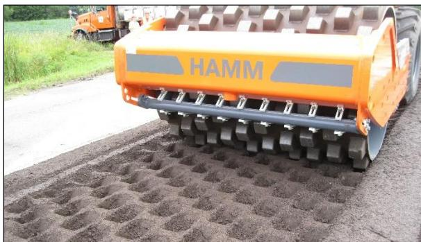
**Figure 6.93: Padfoot impressions after first roller passes (FDR).**
