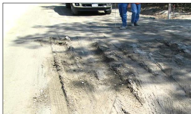
**Figure 6.22: Wet area caused by water leaks during tanker change (FDR).**
