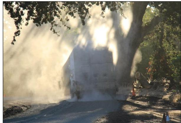
**Figure 6.74: Loss of active filler/stabilizer during windy conditions.**
