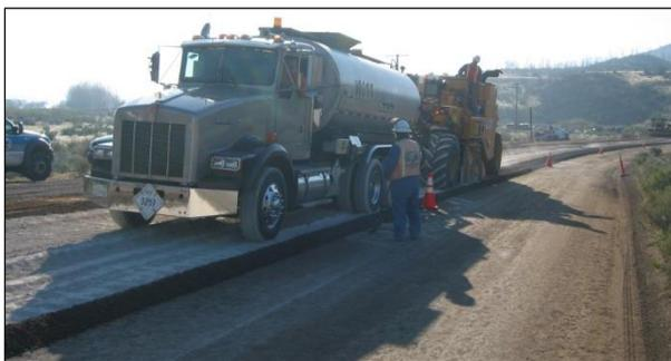
**Figure 6.75: FDR-FA recycling train with no water tanker.**
