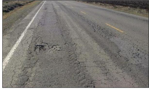
**Figure 2.30: Fatigue cracking and potholes in wheelpath repairs.**
