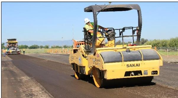
**Figure 6.13: Steel breakdown roller on a PDR layer.**
