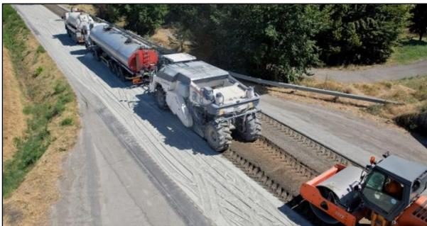
**Figure 6.8: Wheel-driven FDR recycling train.**
