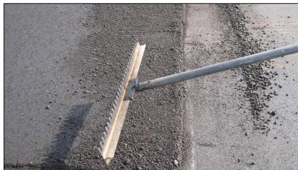
**Figure 6.88: Raking to clear material and provide a sight line for the roller operator.**
