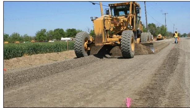
**Figure 6.5: Adding new layer for structural improvement prior to recycling.**
