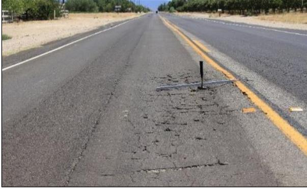
**Figure 2.25: Example bottom-up distresses: Ruts associated with subgrade failure (a).**
