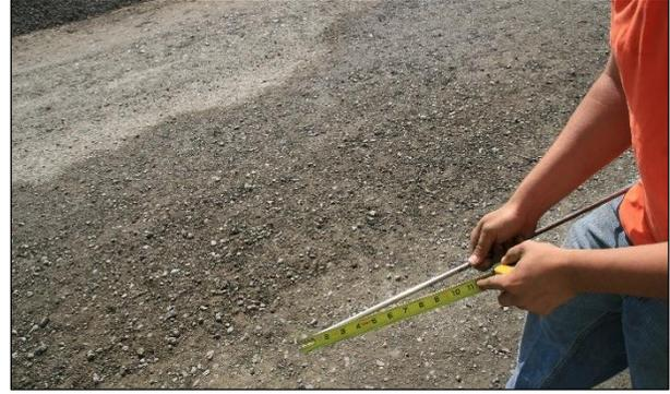
**Figure 6.30: Measuring recycling depth on the T-bar (FDR).**
