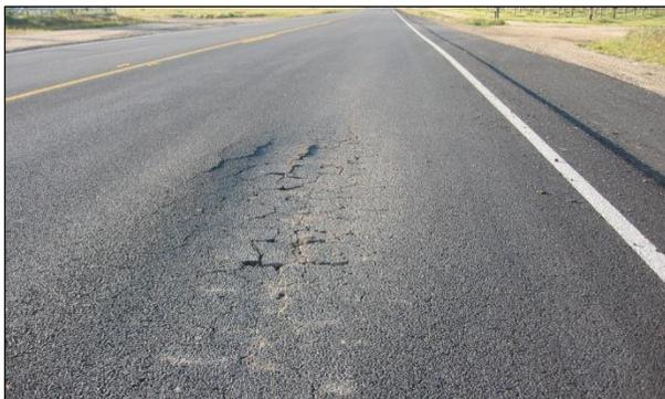
**Figure 6.23: Localized early failure resulting from a wet area (FDR).**
