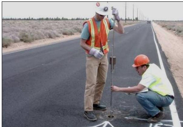
Figure 2.52: DCP test.
