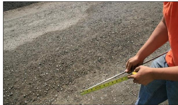
**Figure 6.30: Measuring recycling depth on the T-bar (FDR).**
