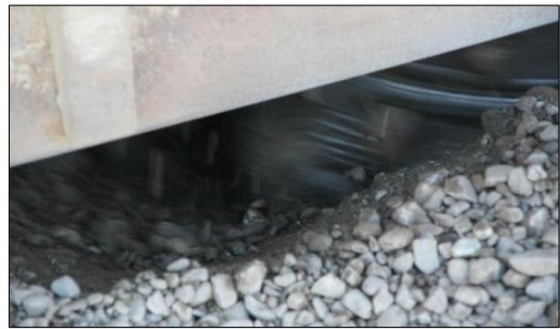
**Figure 6.24: Localized segregation caused by idling recycler drum (FDR).**
