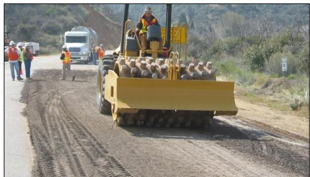
**Figure 6.94: Padfoot impressions after multiple roller passes (FDR).**
