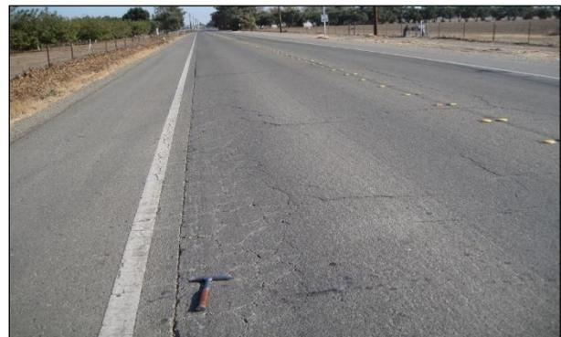
**Figure 6.87: Fatigue cracking in asphalt concrete in the bridged area.**
