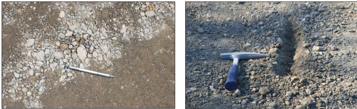
**Figure 6.101: Segregation after excessive movement of material with a grader (FDR).**
