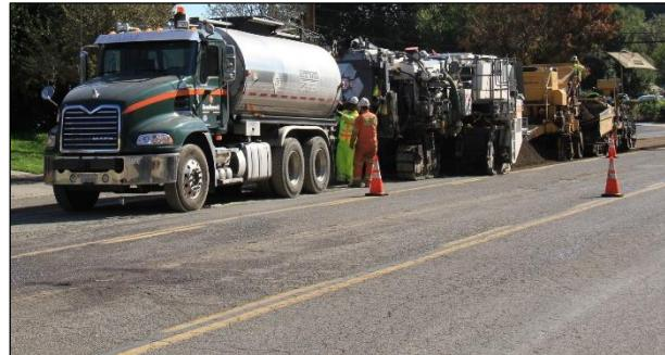
Figure 1.3: Partial-depth recycling train (single unit).
