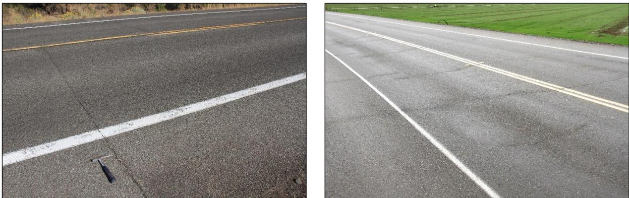
**Figure 3.7: Reflected shrinkage cracks on FDR-C projects.**
