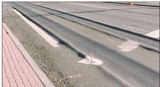
**Figure 2.14: Example top-down distresses: Surface ruts during high temperatures.**
