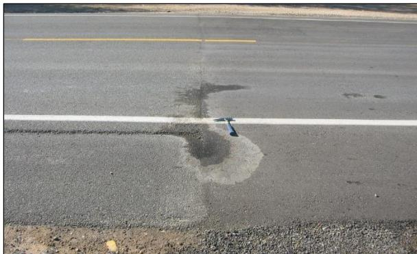
**Figure 2.29: Early failure in patch (note water pumping in join).**
