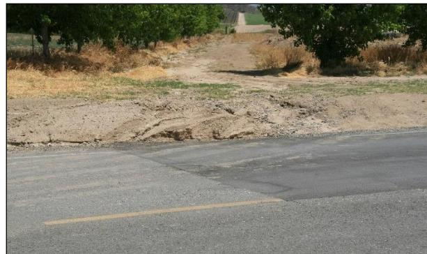
**Figure 2.36: Access road drainage problems (note patch).**
