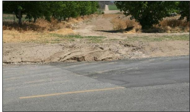
**Figure 2.36: Access road drainage problems (note patch).**
