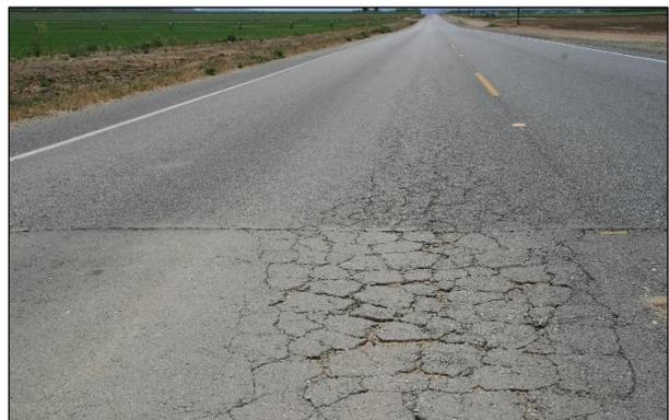
**Figure 2.28: Early failure in patch (drainage problem).**
