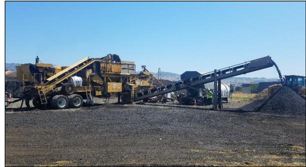
**Figure 6.11: Cold central plant using processing unit from a multi-unit recycling train.**
