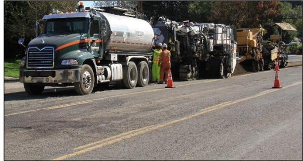
Figure 1.3: Partial-depth recycling train (single unit).
