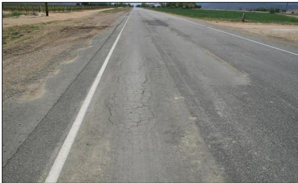
**Figure 2.31: Early failure in wheelpath repairs.**
