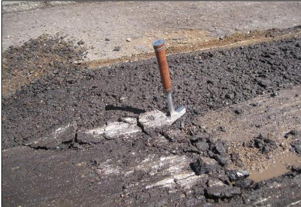
**Figure 6.53: Thin, debonded layer on a PDR project.**
