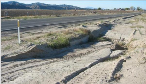
**Figure 2.6: Example blocked side drains and culvert.**
