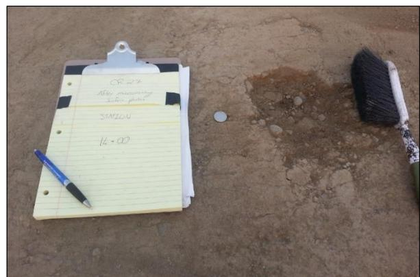
**Figure 6.111: Breakup of surface of an FDR-C layer caused by carbonation.**
