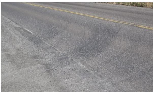
**Figure 6.51: Trafficked recycled layer with no raveling/scuffing from turning vehicles (PDR).**
