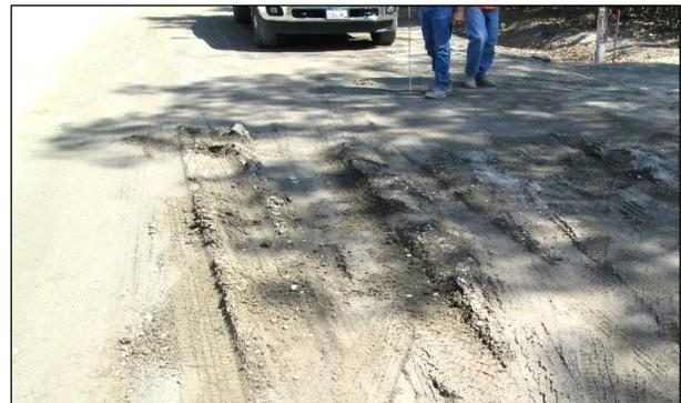
**Figure 6.22: Wet area caused by water leaks during tanker change (FDR).**
