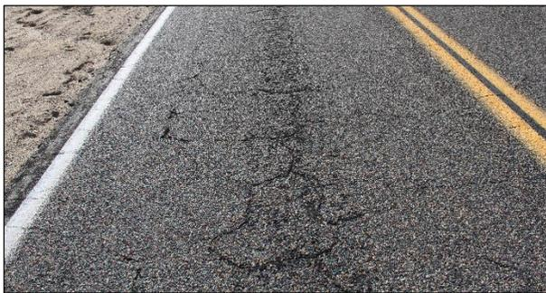
**Figure 2.11: Example top-down distresses: Oxidative aging cracks.**
