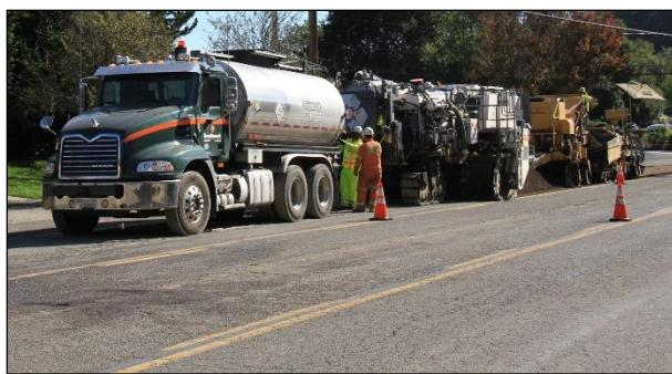
Figure 6.6: Single-unit PDR recycling train.
