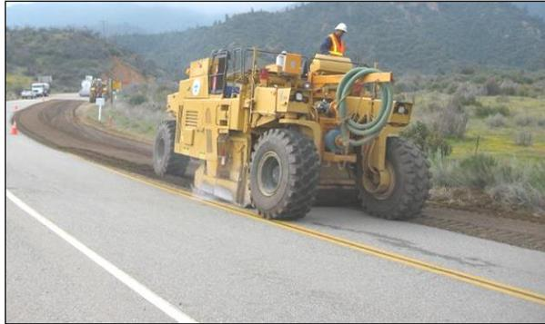
**Figure 6.55: Prepulverization on an FDR project.**
