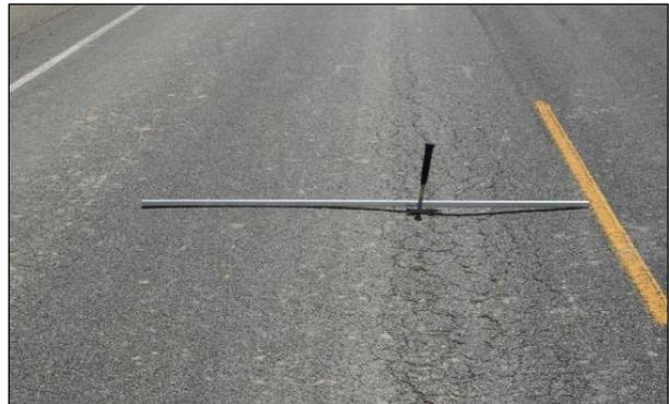
**Figure 2.5: Example rutting associated with base/subgrade failure.**
