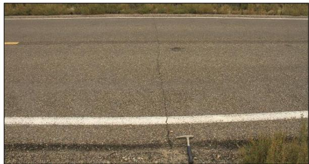
**Figure 2.12: Example top-down distresses: Low temperature thermal cracks.**
