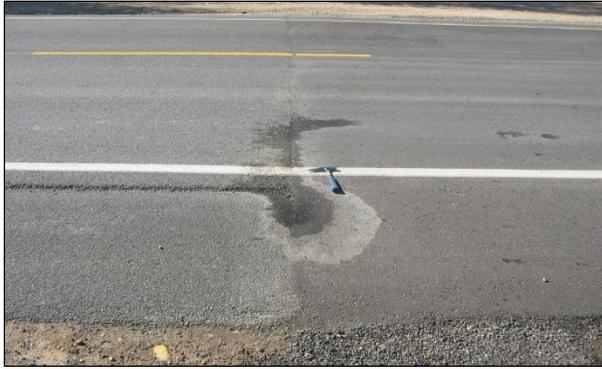
**Figure 2.29: Early failure in patch (note water pumping in joint).**
