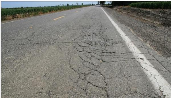
**Figure 6.4: Distressed road prior to addition of new layer.**
