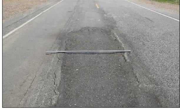
**Figure 2.26: Example bottom-up distresses: Ruts associated with subgrade failure (b).**
