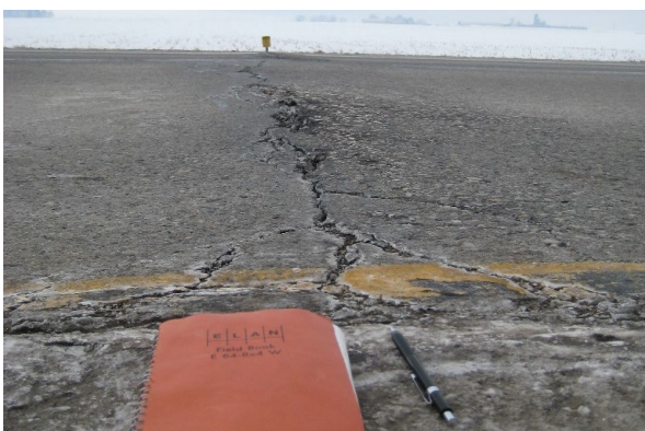
Vertical heave at the joint (air temperature -4°C)
