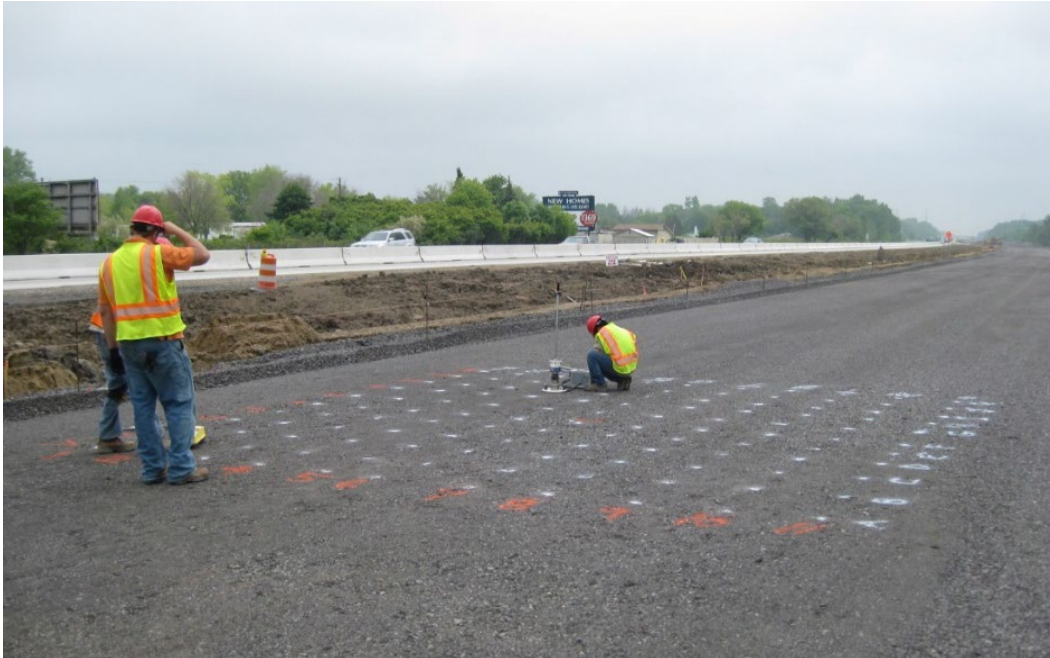
Figure 14. Field testing in a dense grid pattern on an open-graded drainage course granular base layer consisting of recycled steel slag (classified as GP and A-1-a) – Michigan I-94 construction project (photograph taken on May 28, 2009)
