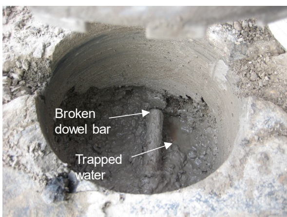
Broken dowel bar and trapped water near bottom of pavement after extracting the core
