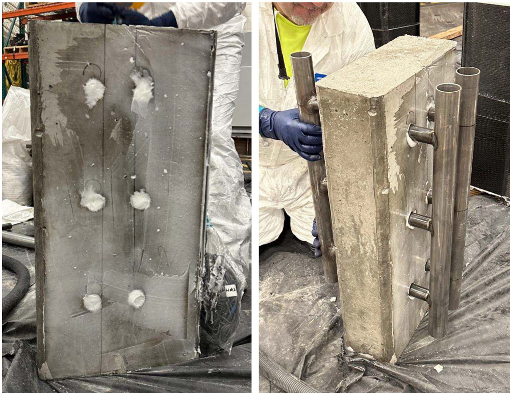
Figure 17 Installation of tubes on columns.
