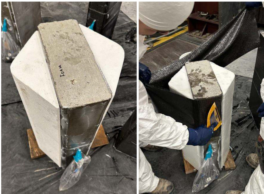
Figure 14 Preparing geofoam-profiled FRP jacket.
