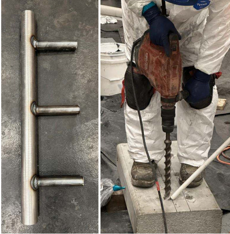
Figure 16 Steel-tube and preparation of columns.
