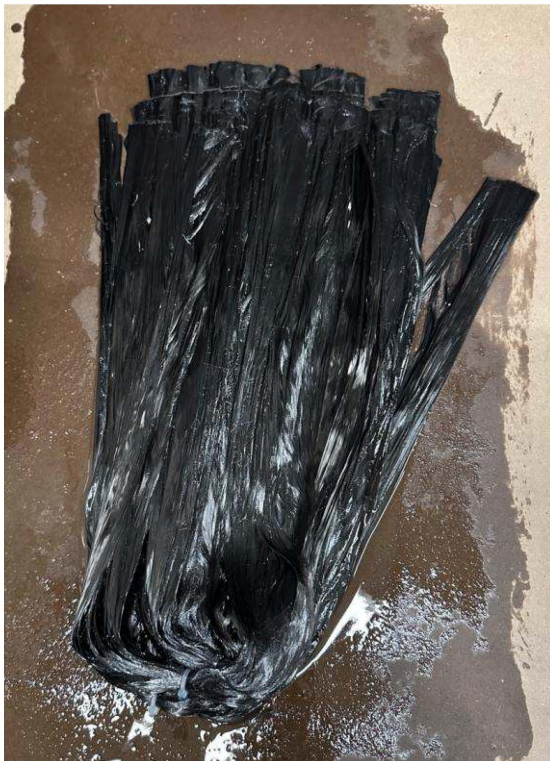
Figure 12 Preparing FRP anchor with resin.
