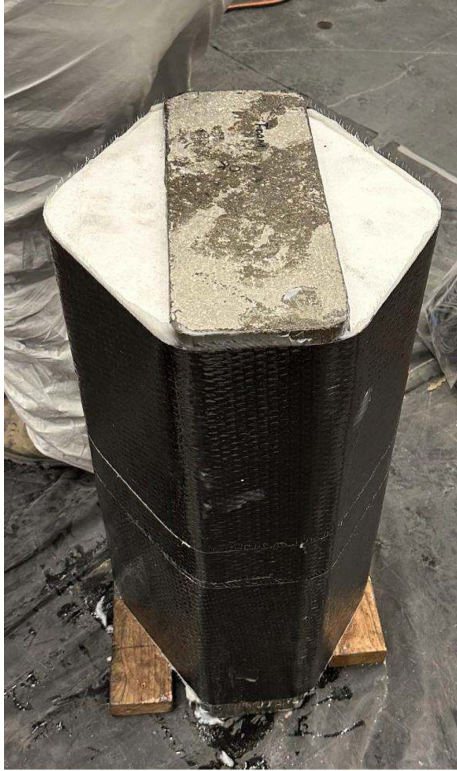
Figure 15 Columns with geofoam-profiled FRP jacket.
