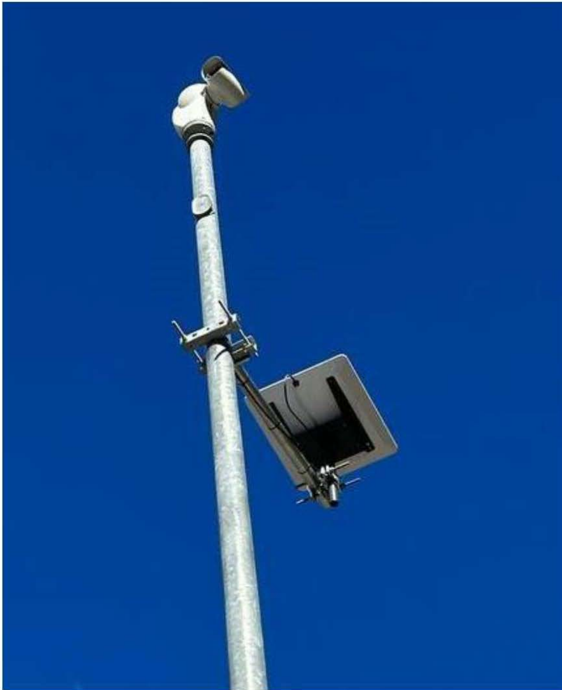
Figure A.16: Second view of a complete Starlink Ground Pole installation at a field site
