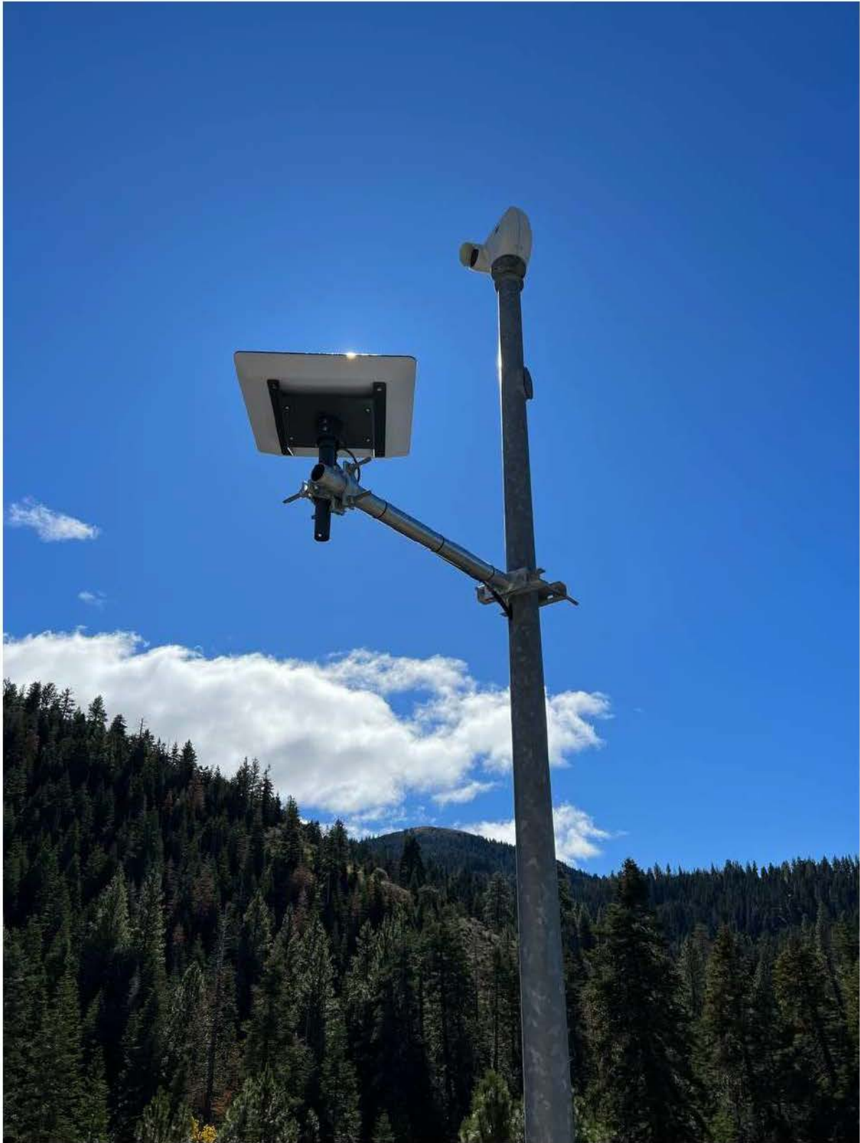
Figure A.15: First view of a complete Starlink Ground Pole installation at a field site
