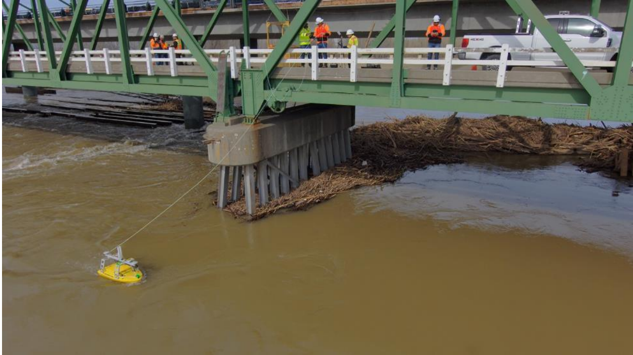
Figure 3.7: EchoBoat-160 Survey emergency pilot project in turbulent water at Butte City Bridge over Sacramento River. Image courtesy of Caltrans.
