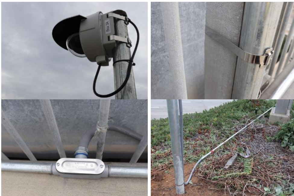
Figure A1.7: Details of camera mounting and cabling at Las Flores Overcrossing
