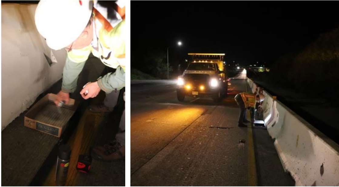
Figure 2.10: Road marking application with spray paint
