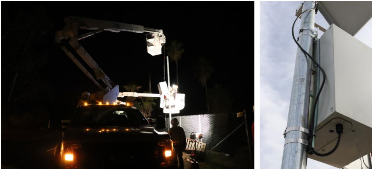
Figure A1.8: Left: Installation of electronics box at Jefferson Overcrossing with a bucket truck. Right: Straps around the steel pole
