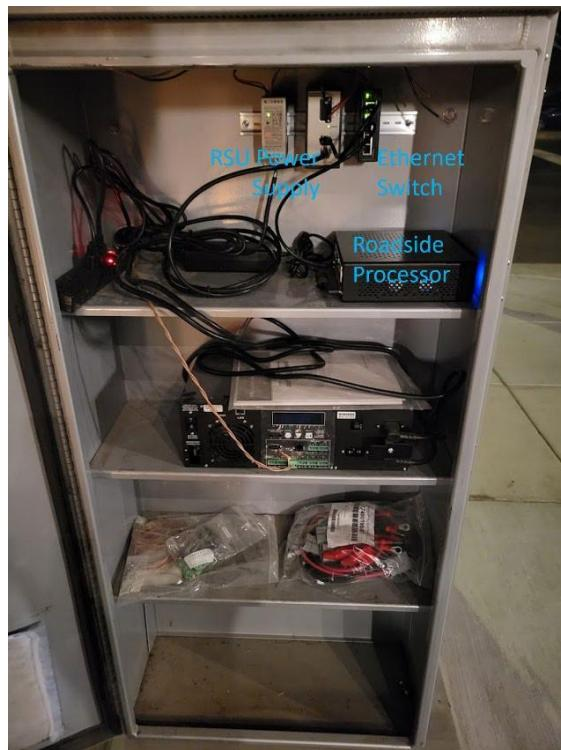
Figure 9 CV Equipment inside the Backpack Cabinet
