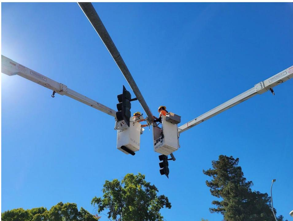
*Figure 7 Mounting the RSU on the Mast Arm
