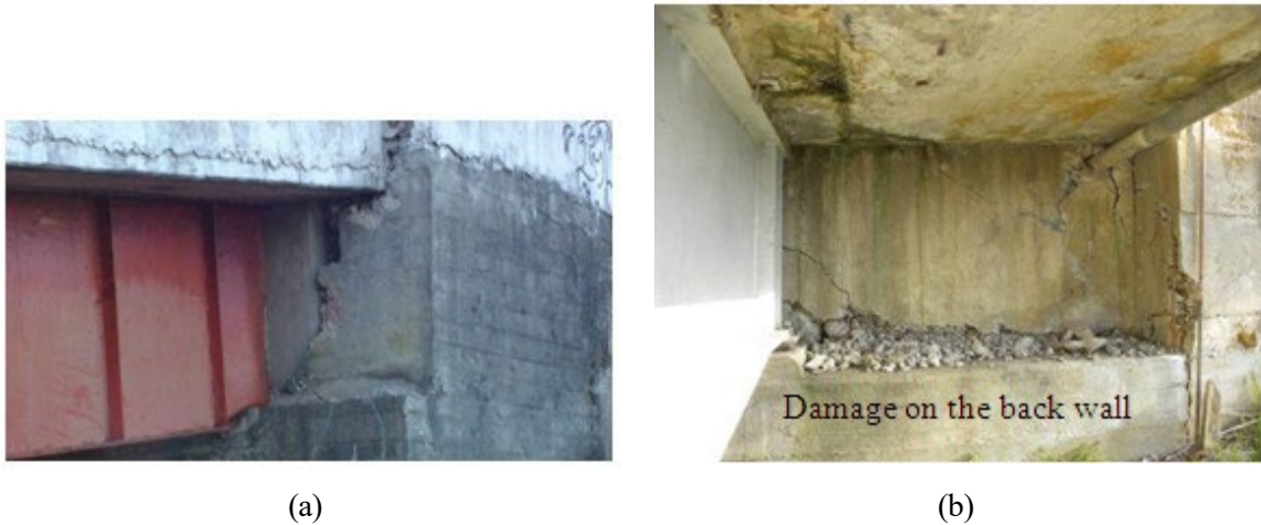
Figure 2.8: Examples of backwall damage (Jibson and Harp, 2011): (a) punching of the Tubul bridge deck into the backwall of the north abutment, and (b) damage at the base of the north abutment backwall of the El Bar bridge.
