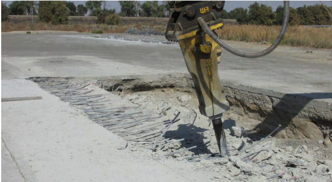
Figure 2-2 Top 12 Inches of Concrete Being Removed from Anchor Block
