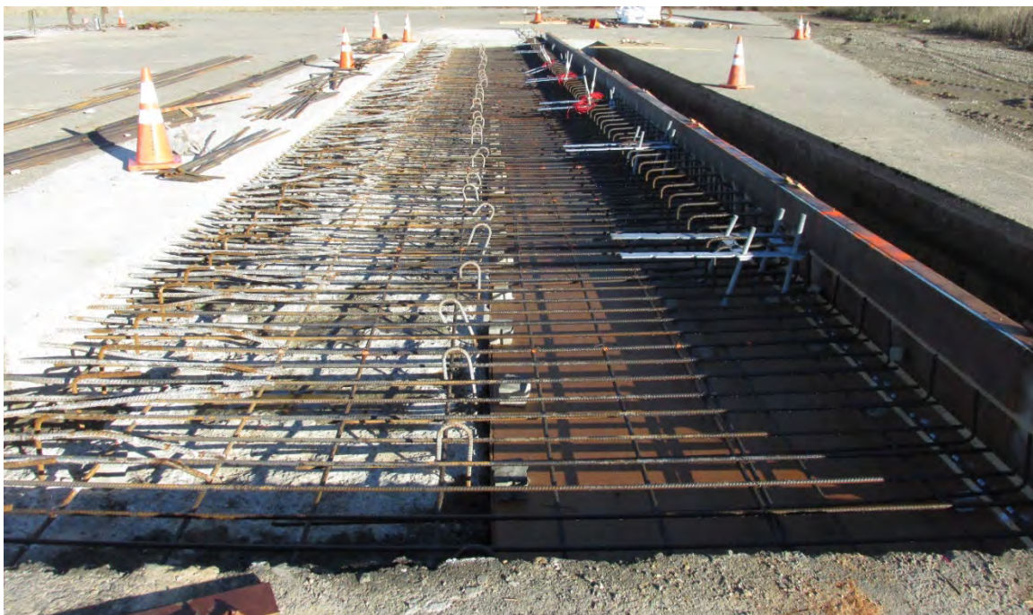
Figure 2-3 Rebar and Strain Gauges in Place for Anchor Block Concrete Replacement and Deck Overhang
