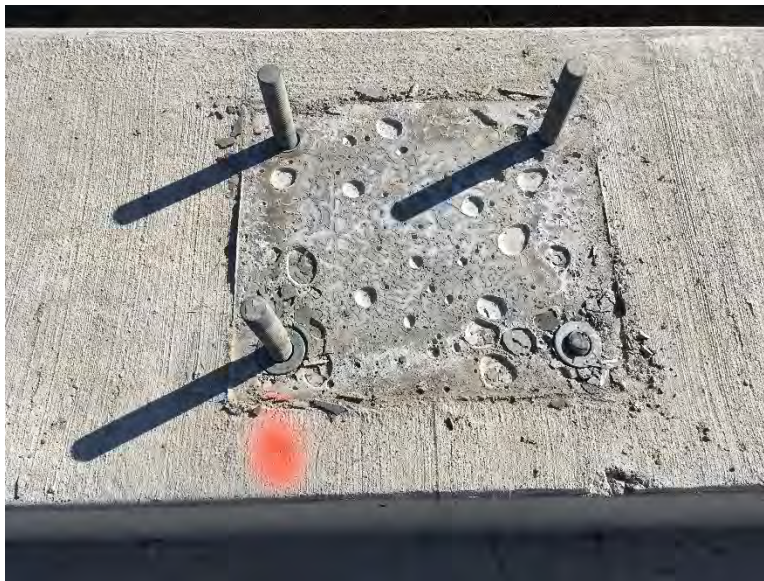
Figure 11-4 Post 6 Anchor Bolts with Post Removed
