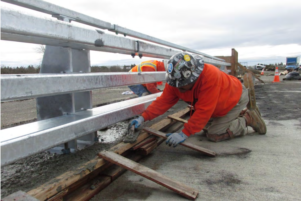
Figure 2-10 Bridge Rail Curb Concrete Pour
