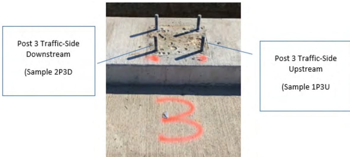
Figure 11-2 Post 3 Anchor Bolts with Post Removed
