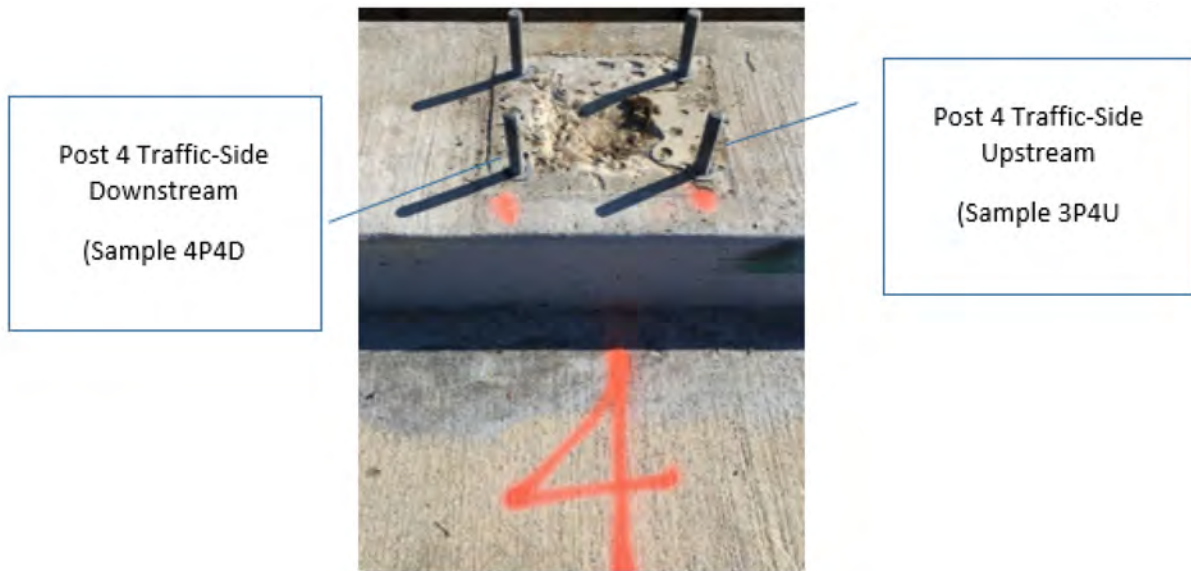
Figure 11-3 Post 4 Anchor Bolts with Post Removed
