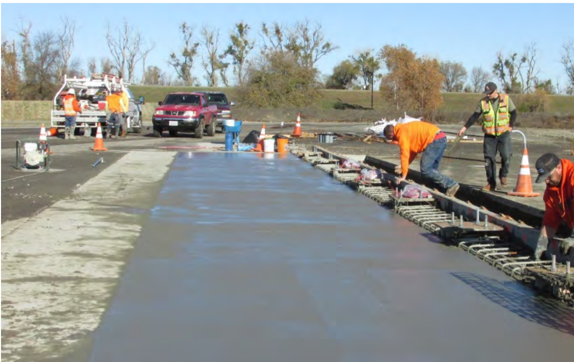
Figure 2-9 Simulated Deck Concrete Pour Complete
