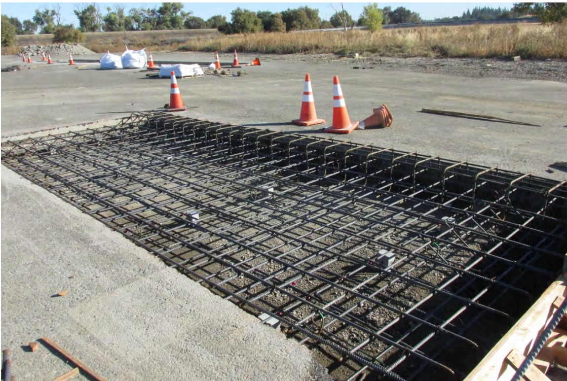
Figure 2-5 Rebar in Slab Footing for Downstream Section
