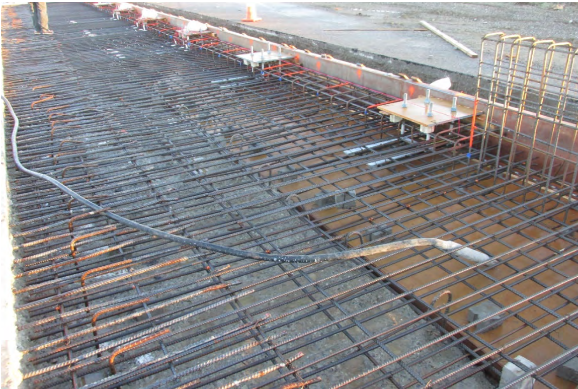
Figure 2-7 Reaction Block and Deck Rebar in Place for Concrete Pour
