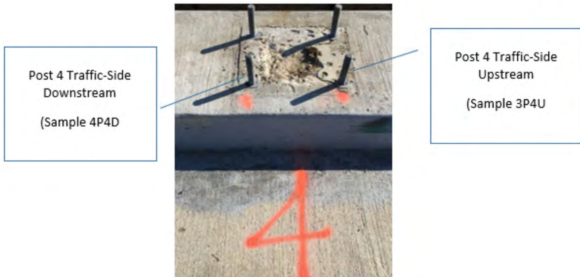
Figure 11-3 Post 4 Anchor Bolts with Post Removed
