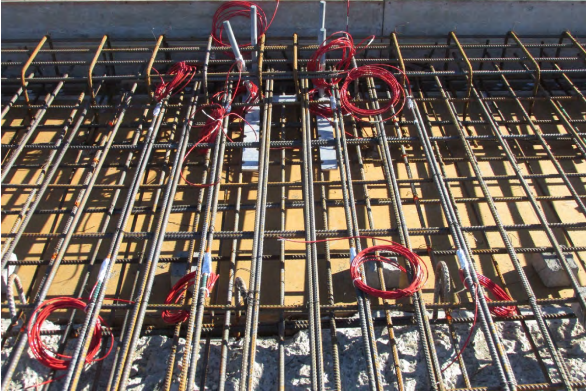
Figure 2-4 Uniaxial Strain Gauges and Cable Prior to Deck Pour
