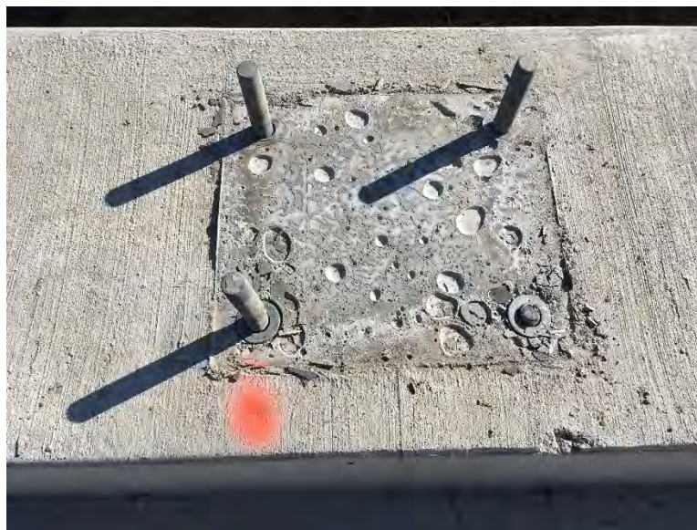
Figure 11-4 Post 6 Anchor Bolts with Post Removed
