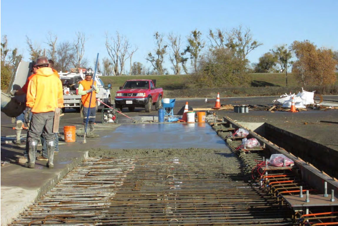
Figure 2-8 Formwork and Rebar in Place for Simulated Deck Concrete Pour
