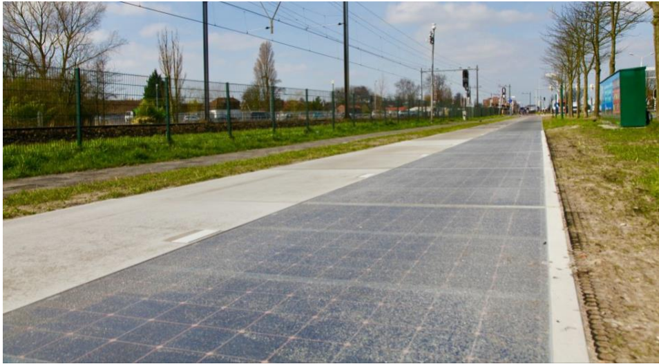
Figure 3. The SolaRoad project in the Netherlands.
