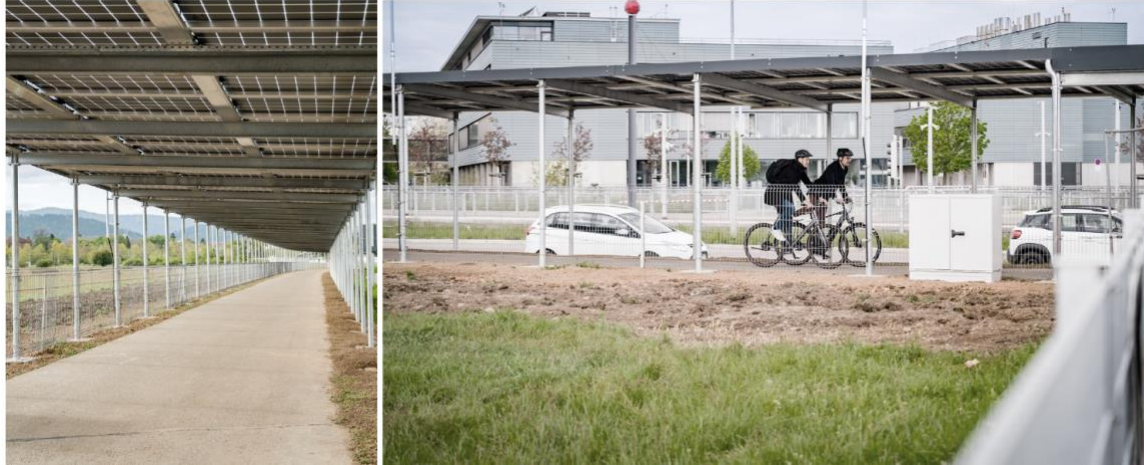
Figure 1. Solar cycle path roofing in Freiburg, Germany.
