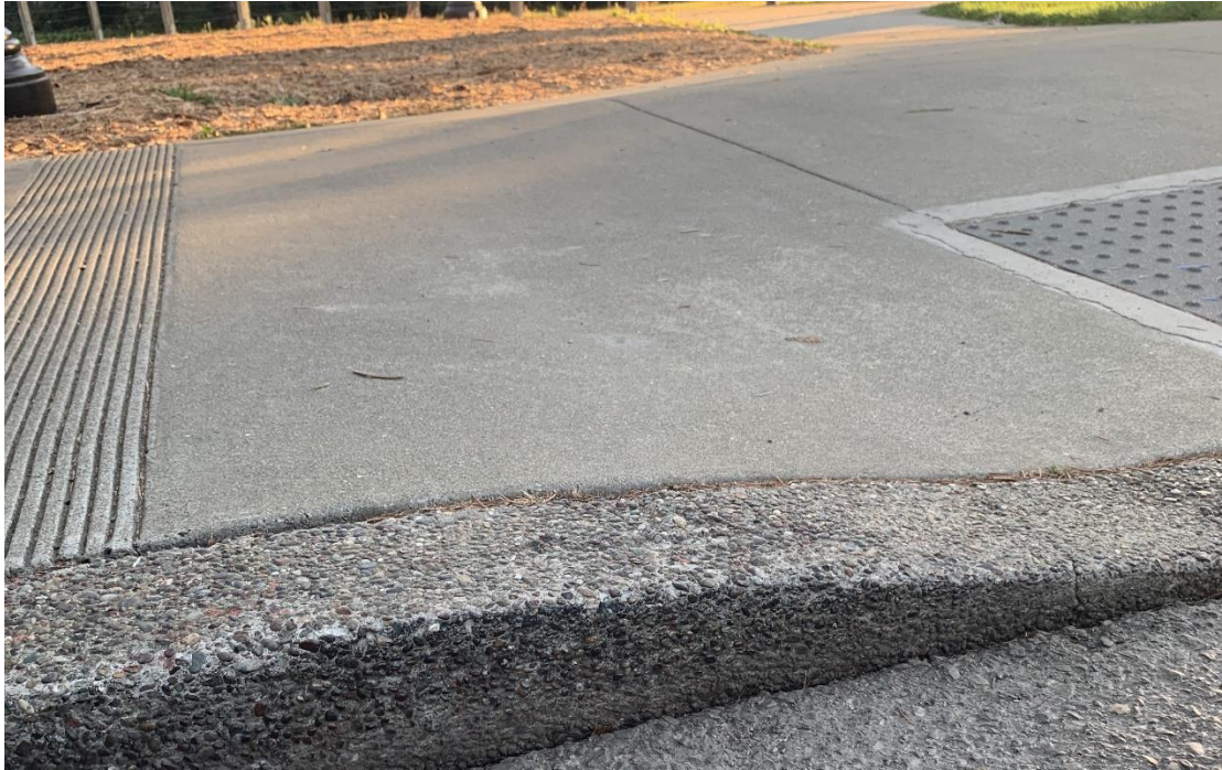
Figure 3.4: Photo of a side flare. The visual features often do not overlap with geometric attributes, and the deviations can be significant.
