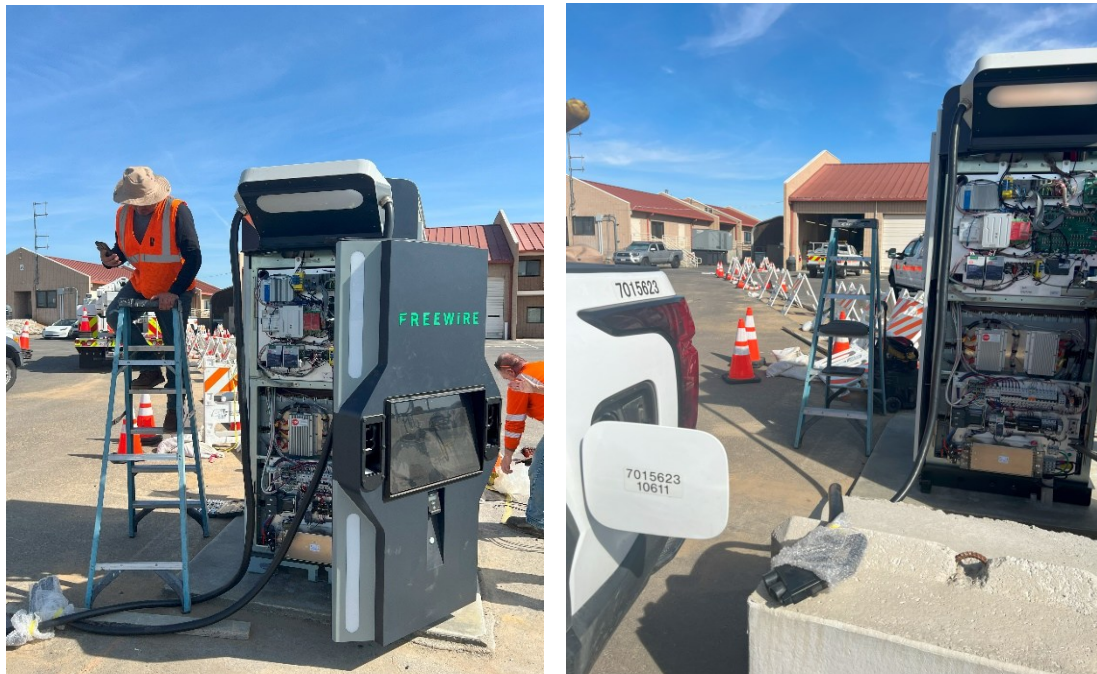
Figure 3.13: Photos showing final commissioning of FreeWire Boost Charger 200
