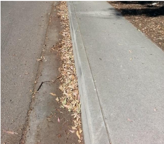
Figure 6.19: Example of area with too much debris that would obstruct MTLs feature extraction.
