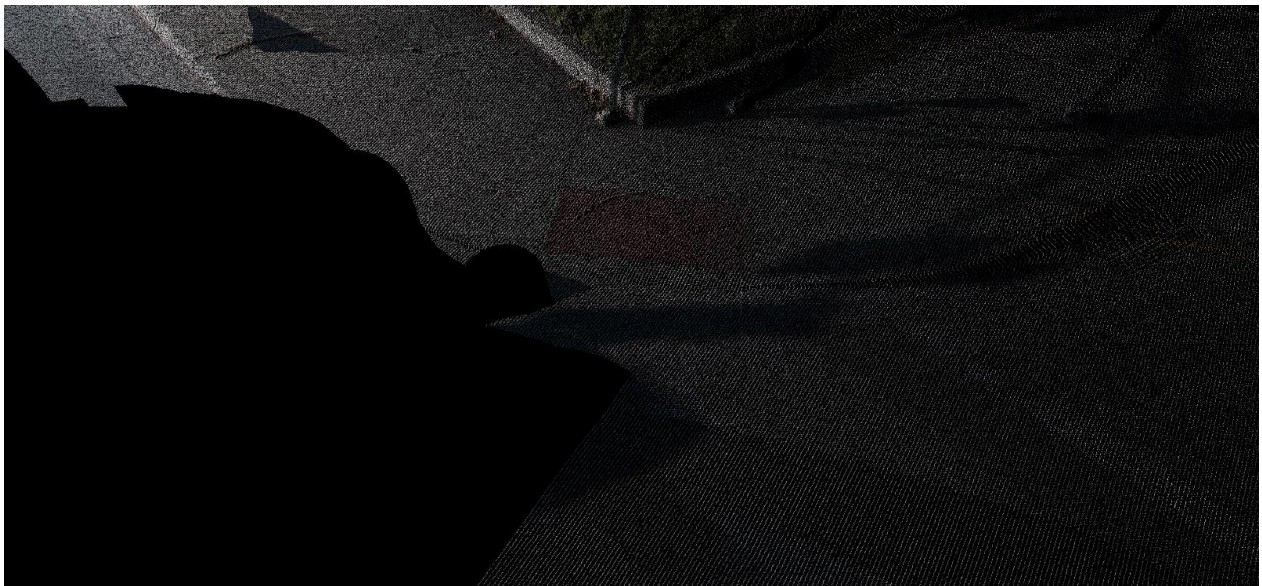
Figure 6.17: Example ADA ramp point cloud with shadow (point data void) caused by vehicular traffic.
