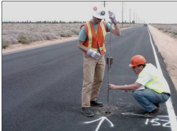
Figure 3.48: DCP testing (manual DCP).
