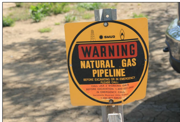
Figure 2.12: Example of gas pipeline warning sign on side of road.
