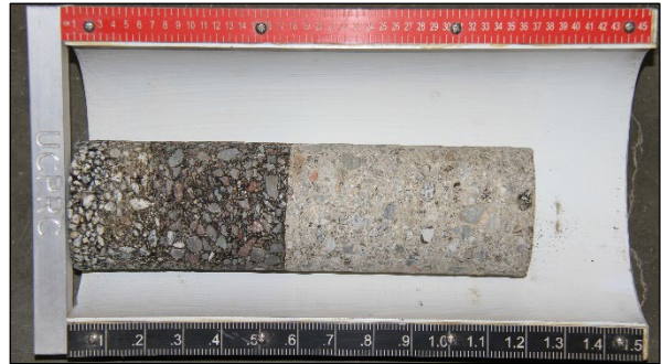
Figure 3.40: Core with asphalt concrete surface over cement concrete (layers are bonded).
