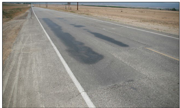
Figure 3.35: Bleeding in digout repairs.
