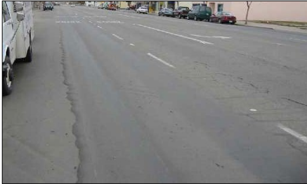
Figure 3.9: Asphalt concrete rutting (top 2 to 4 in., with hump at side of wheelpath).
