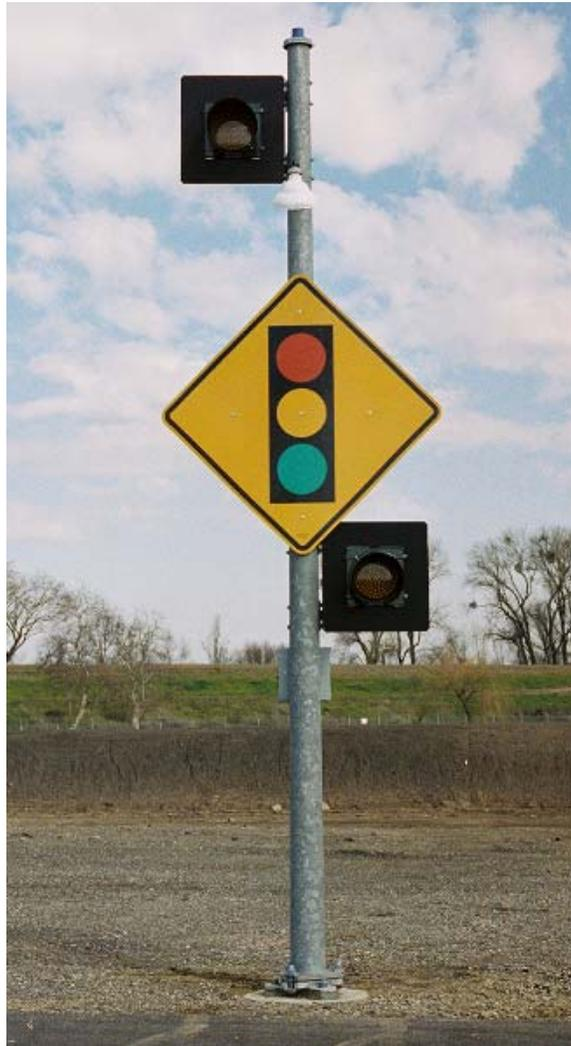
Figure 2-5. Warning Sign with Flashing Beacons
