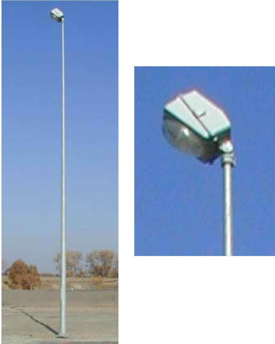
Figure 2-6. Pole Top-Mounted Luminaire (Overall View and Close-Up View of Head).
