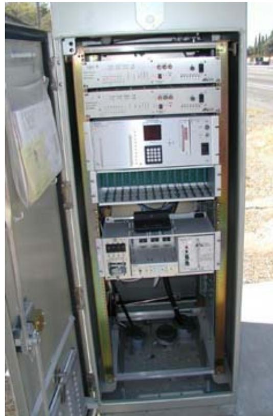
Figure 2-2. Type 334C Controller Cabinet Configured for Onramp Metering
