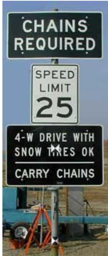
Figure 2-4. Rotatable Chain Control Sign
