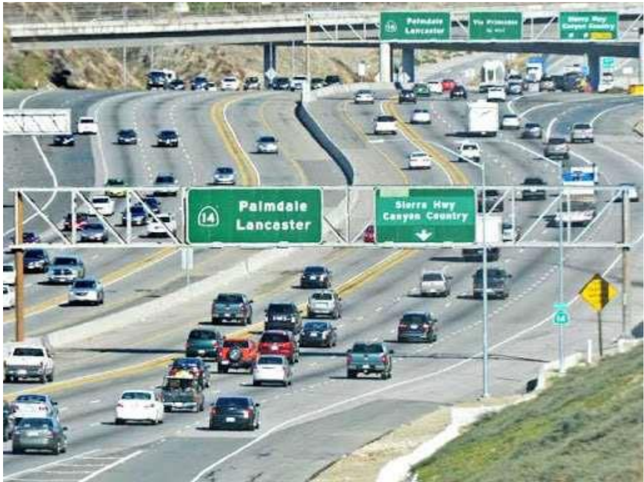
Figure 48. SR-14 with single HOV lane in each direction
