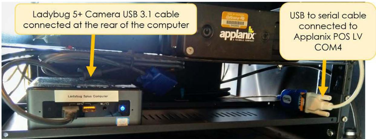
**Figure 5.6: Ladybug 5+ data collection computer setup**
