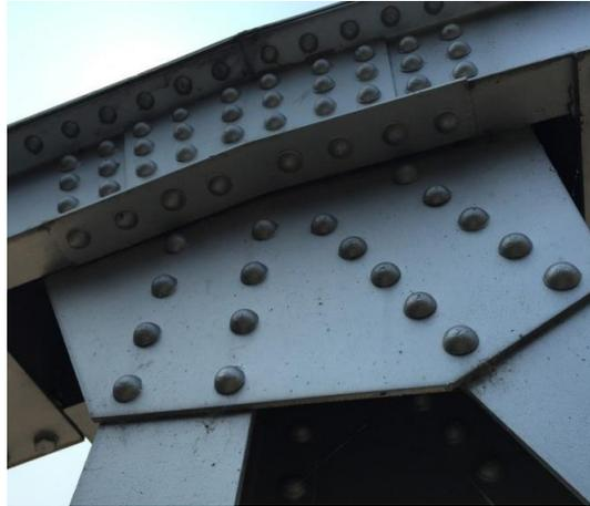
Figure 4.5 Gusset Joints at U2
