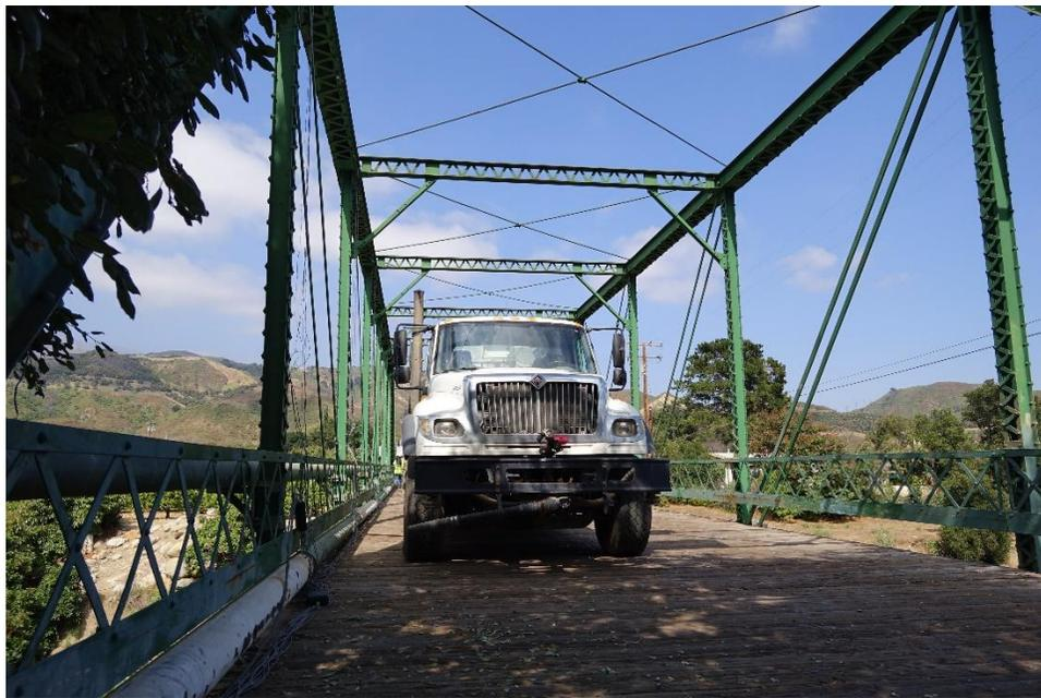
(b) Positioning of Water Truck for Load Test
