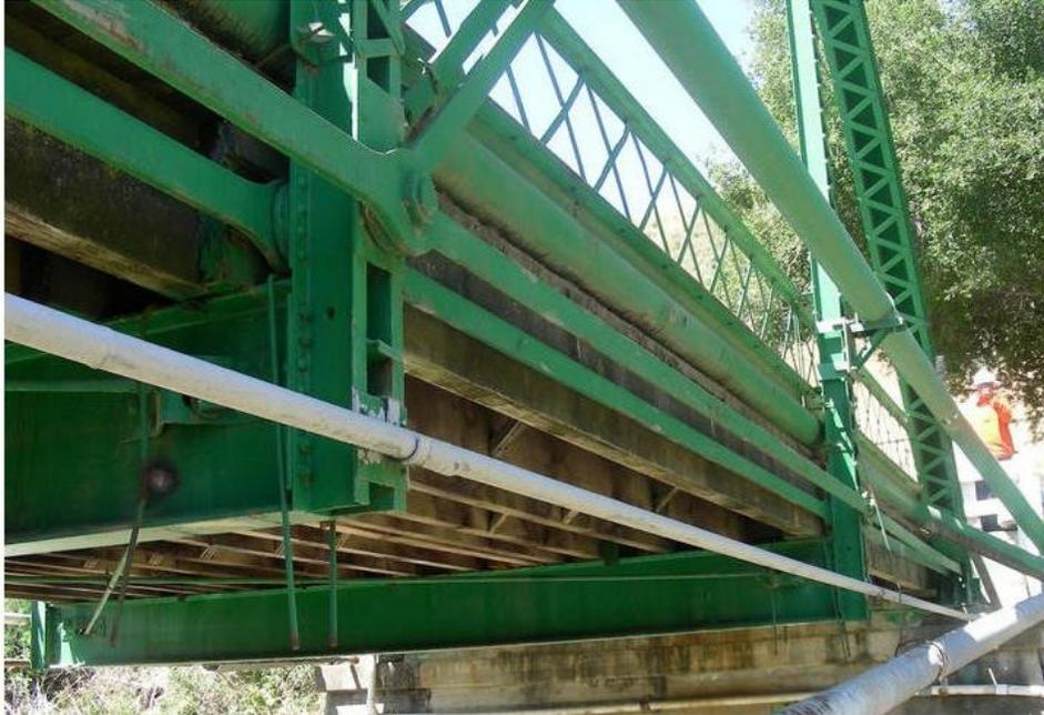
Figure 2.4 Pin-connected Eyebars (Bottom Chord and Diagonal Brace)
