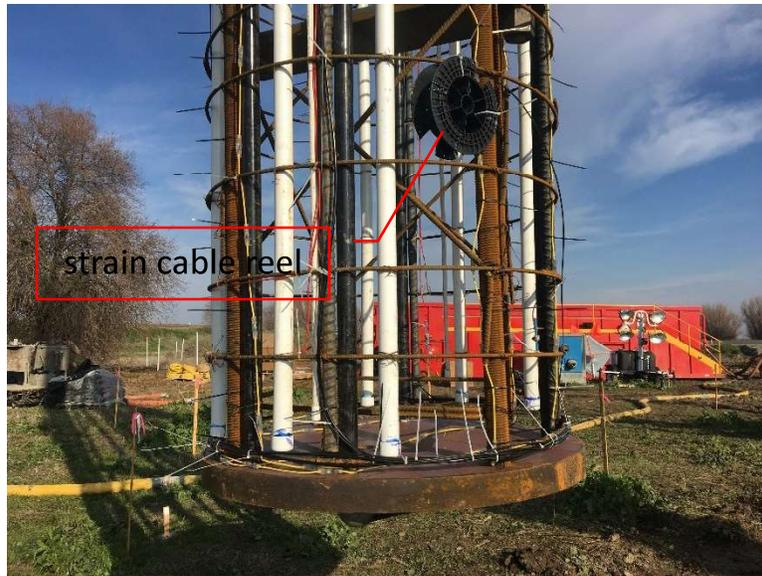
*Figure 4-15: Cable reel attached to the bottom of the cage on vertical inaccessible when cage was on the ground*
