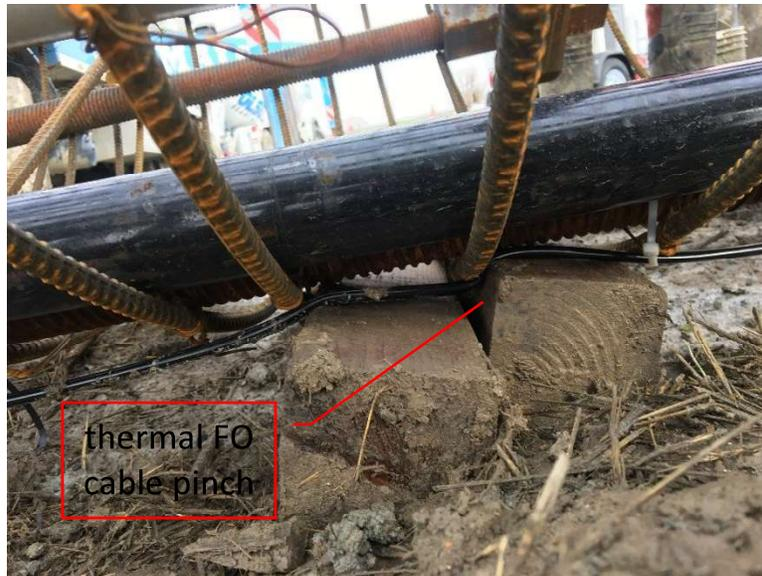
*Figure 4-22: Thermal fiber optic cable pinched under reinforcement during handling prior to installation*
