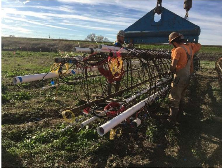
*Figure 4-14: All instrumentation wiring installed and coiled, cage prepared for final pick*
