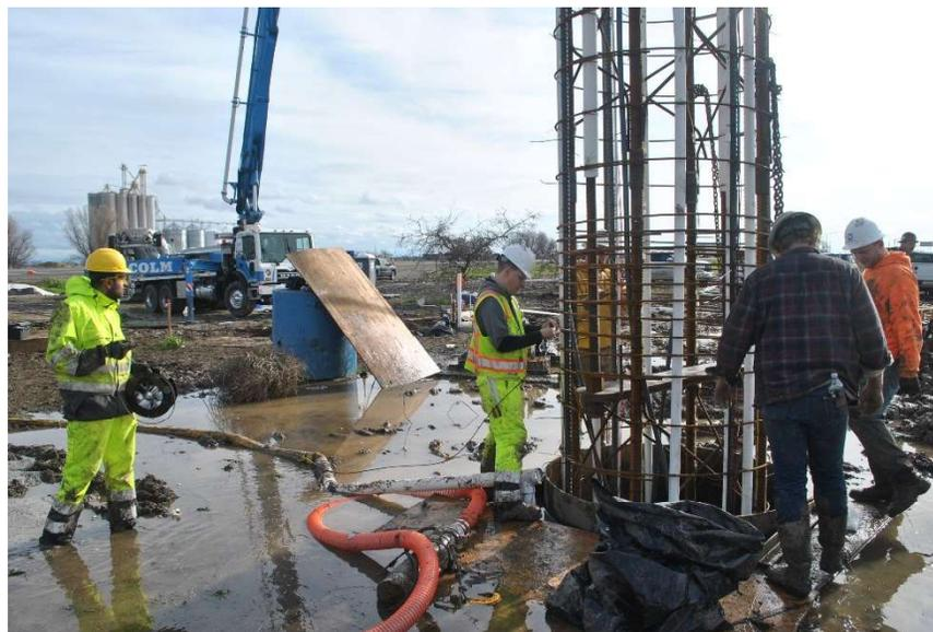
*Figure 4-16: Installation of final fiber optic cable vertical during lowering of reinforcement cage*
