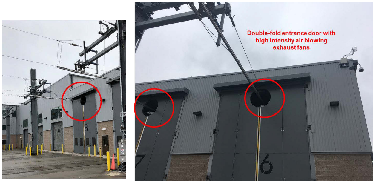
Figure 38: Double-fold entrance door with high intensity air blowing exhaust fans
