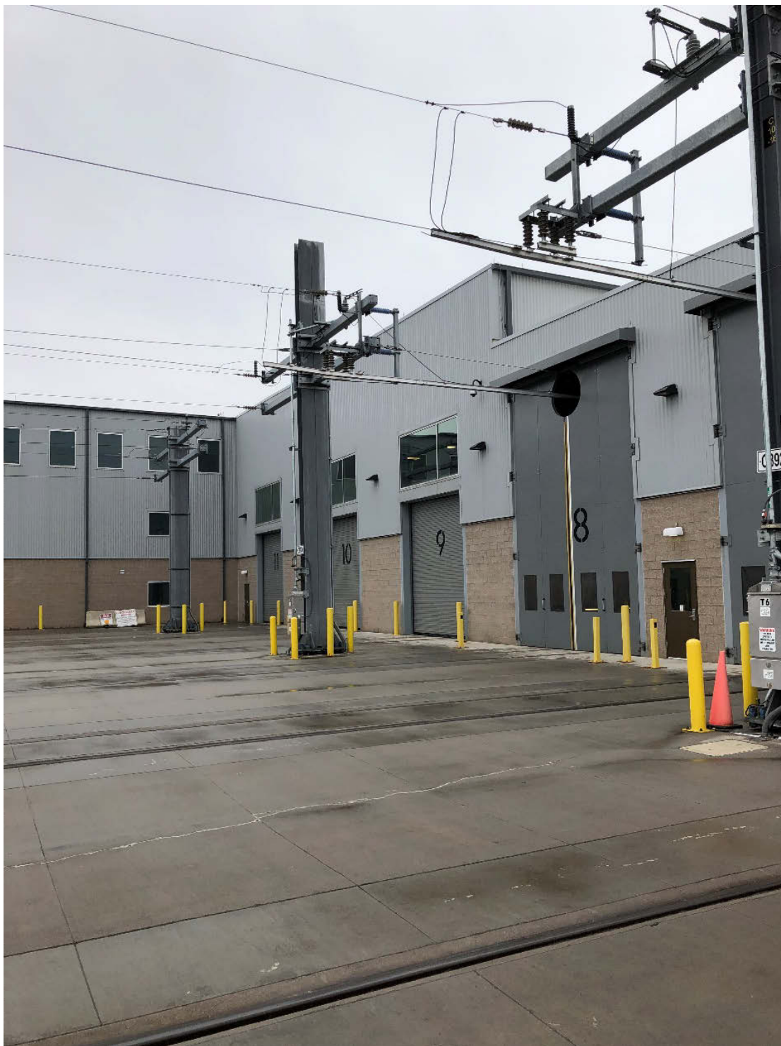
Figure 35: The facility's doors – Roll-up aluminum doors for regular tracks and tall double-fold steel doors for powered tracks
