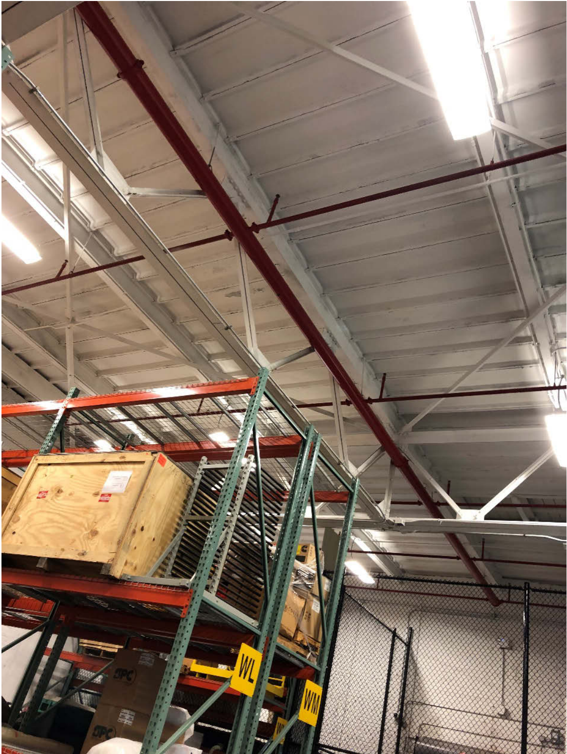
Figure 49: Two-way truss-joists supporting roof steel beams – Materials storage building
