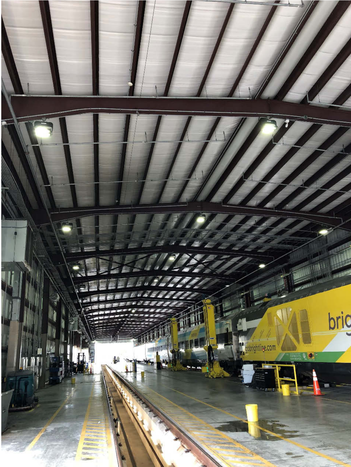
Figure 44: Building structural components: steel portal frame, concrete slab on grade, and the maintenance pit
