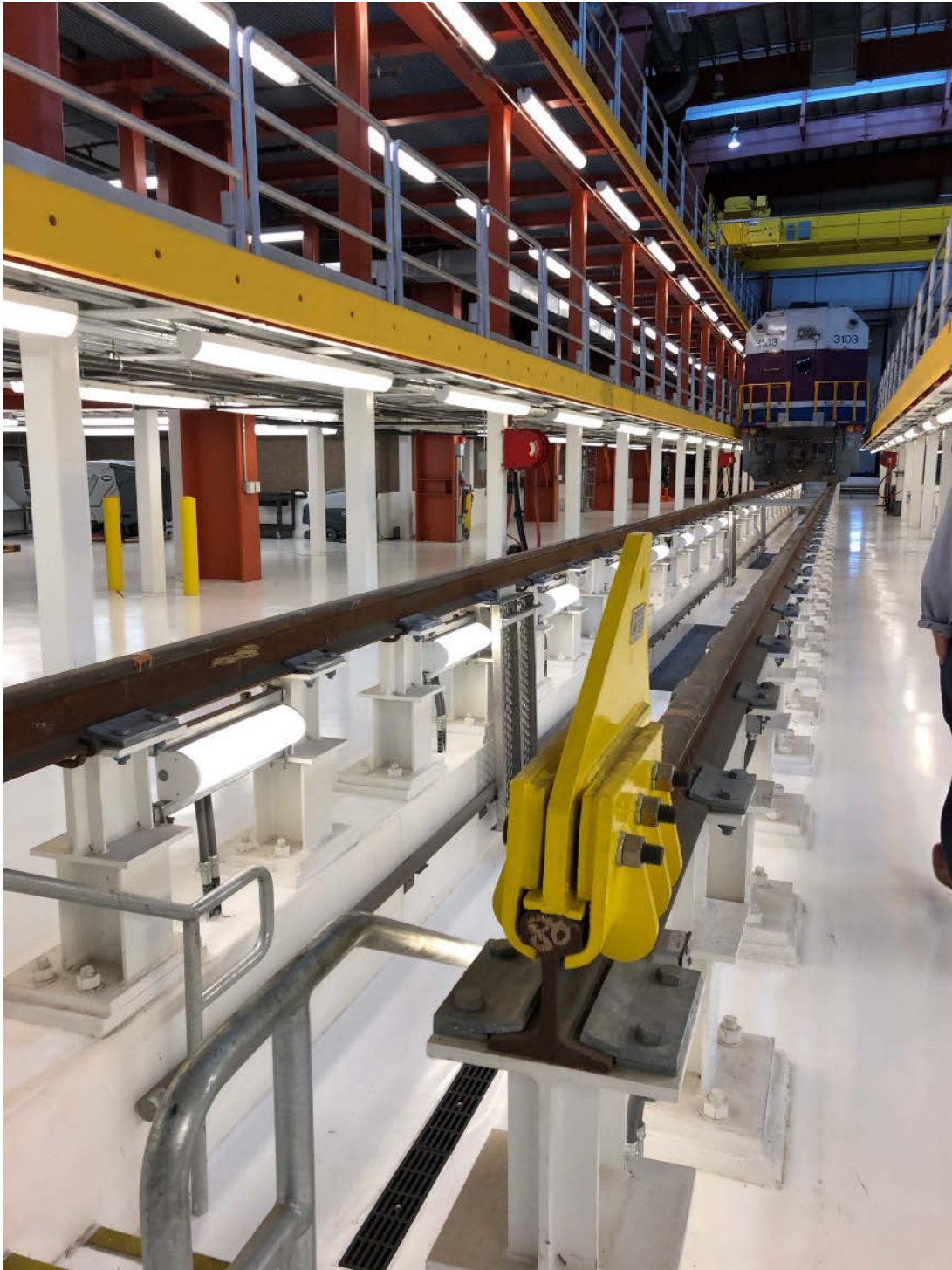
Figure 19: Raised steel deck flooring seated on steel HSS columns and the raised track supported on H-shape steel piers
