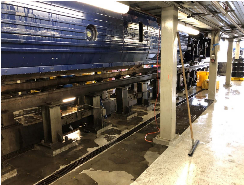
Figure 11: Raised steel deck flooring on steel HSS columns and the raised track supported on H-shape steel piers
