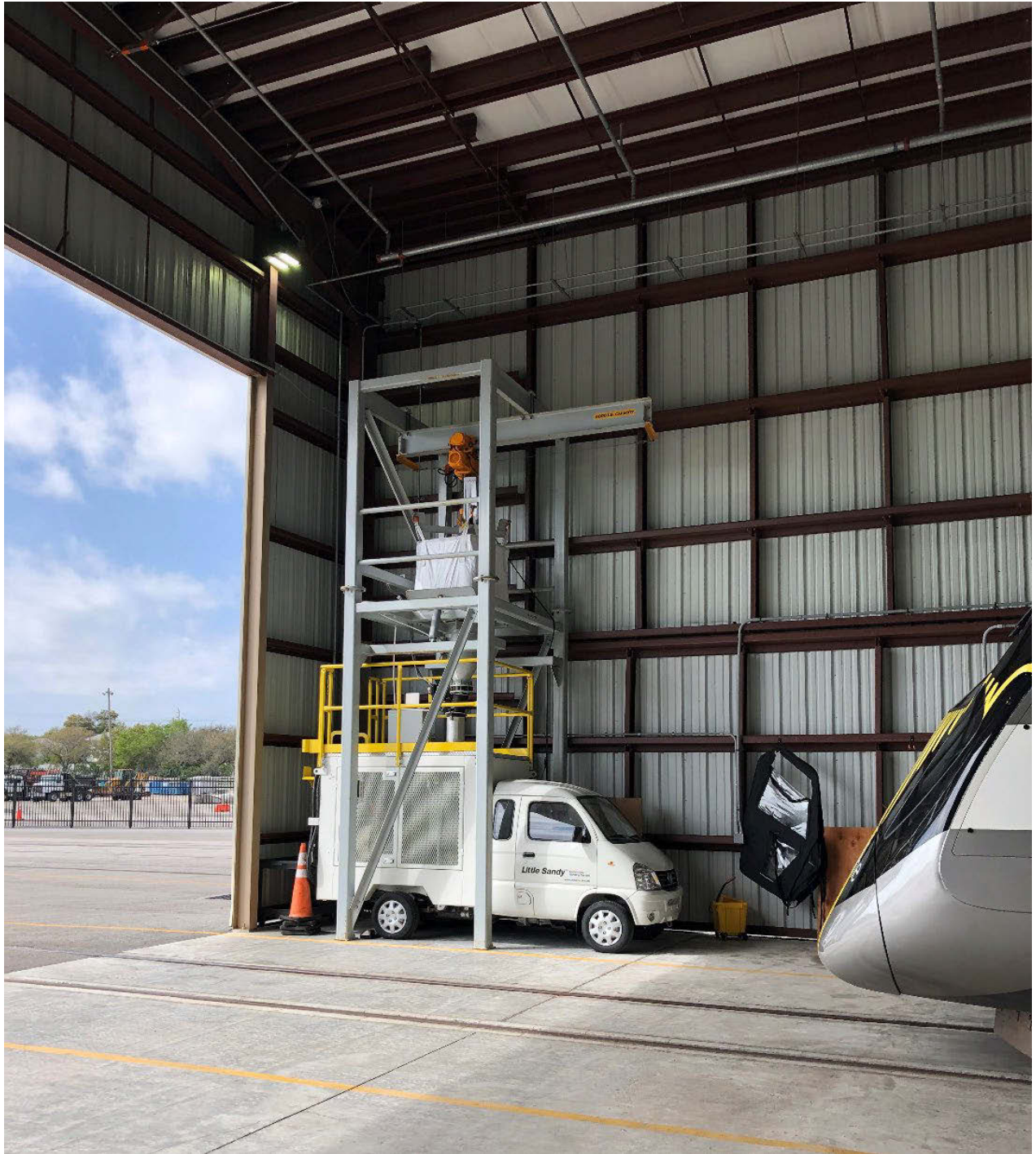
Figure 45: Maintenance building's perimeter enclosure: horizontal steel braces and vertical studs and attached corrugated metal sheets
