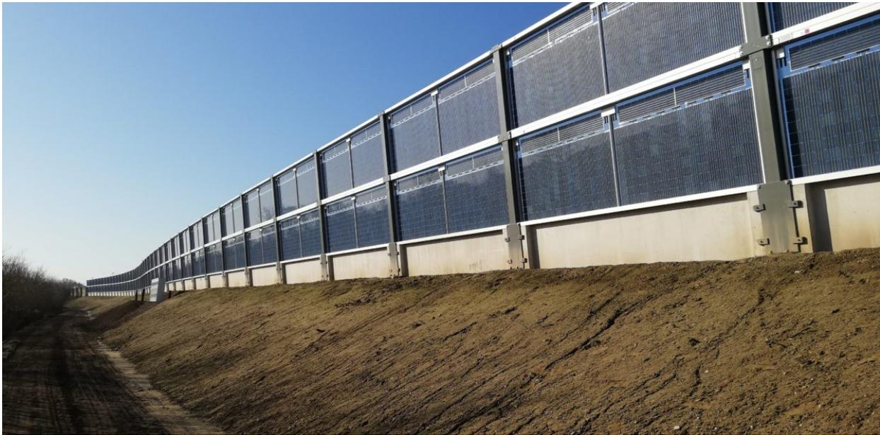
**Figure 3.1. Bifacial modules for noise barriers.** Image source: Solar Energy Application Centre, <https://www.pv-magazine.com/2019/02/20/bifacial-modules-riding-down-the-highway/>.
