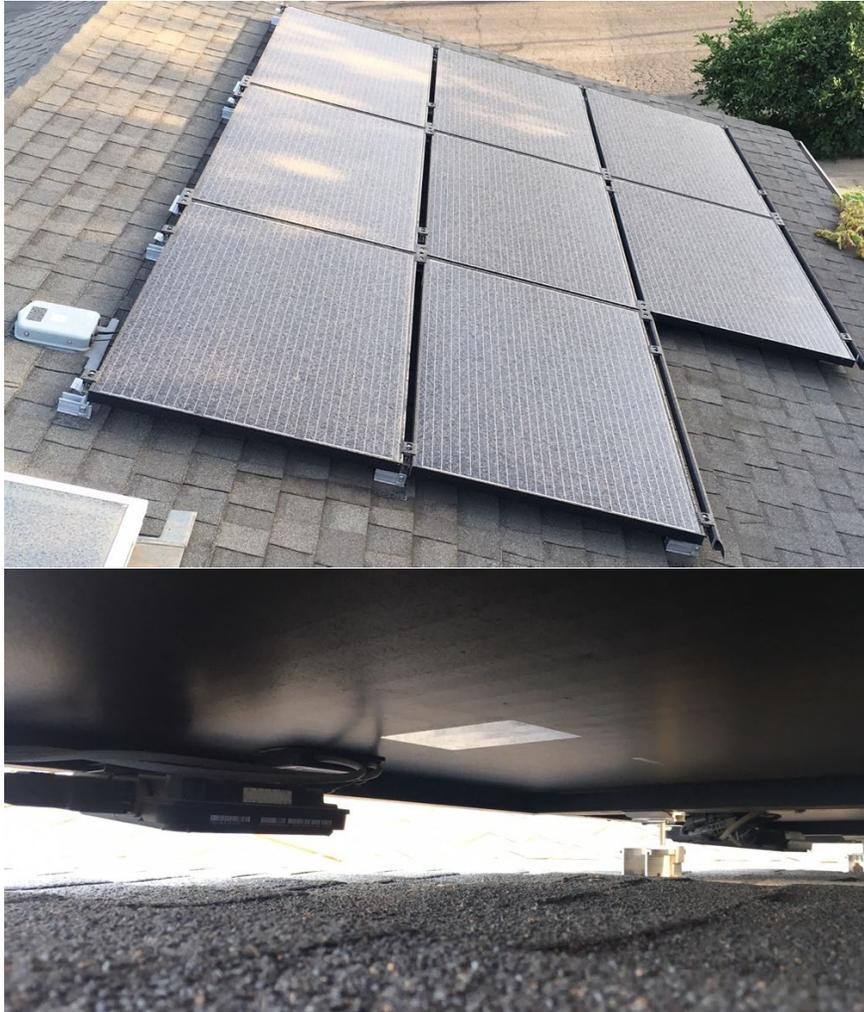
**Figure 6.21. System with microinverters (top); microinverter between module and roof (bottom).**
