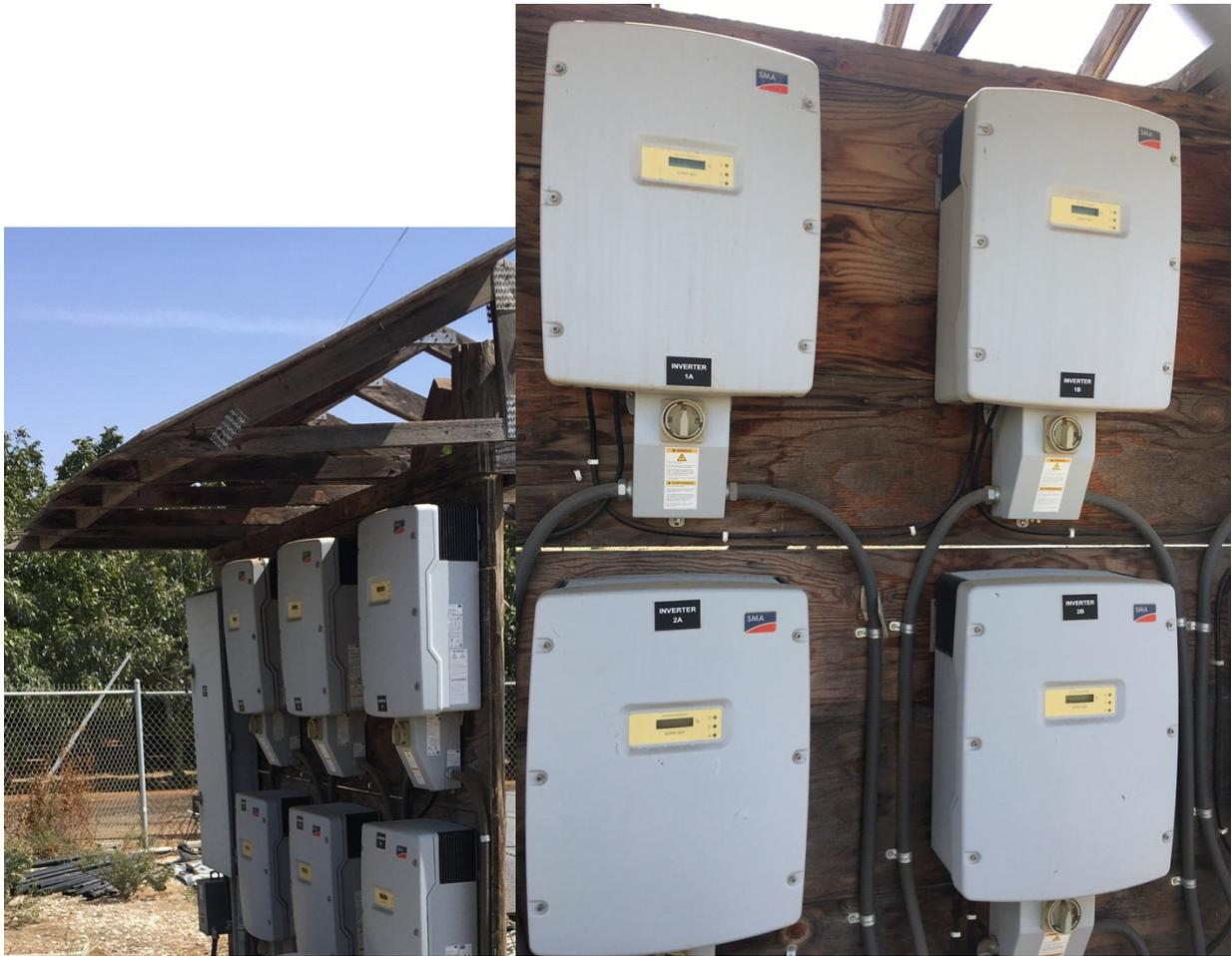
Figure 6.20. SMA string inverters. Photo credit: Kurtz.
