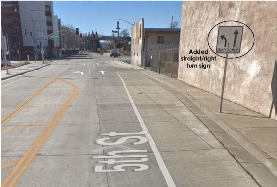
Figure 4.38: Caltrans' sign addition for southbound 5<sup>th</sup> Street on the north side of the intersection at the South River Road exit ramp. Image courtesy of Google Street View.
