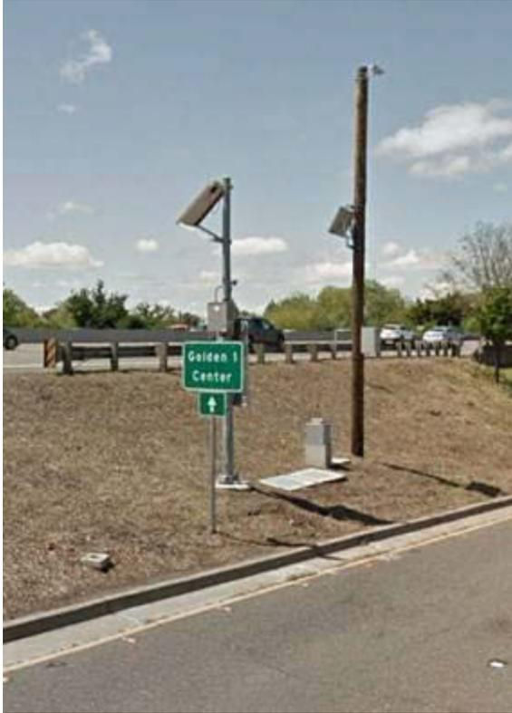
**Figure 4.41: TAPCO radar sensor blocked by informational sign for the 16<sup>th</sup> Street exit ramp system. The AHMCT VBSM can be seen behind the TAPCO system.**
