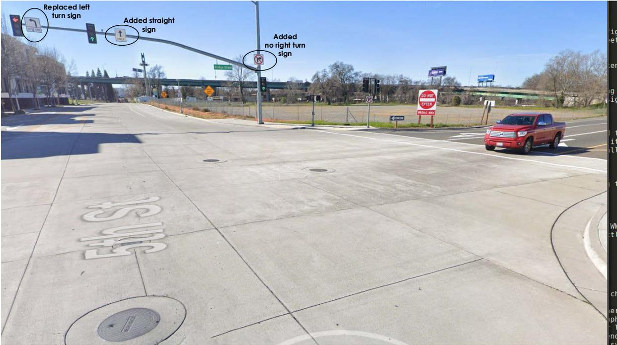
Figure 4.39: Caltrans' sign modifications and additions for southbound 5<sup>th</sup> Street on the south side of the intersection at the South River Road exit ramp. Image courtesy of Google Street View.
