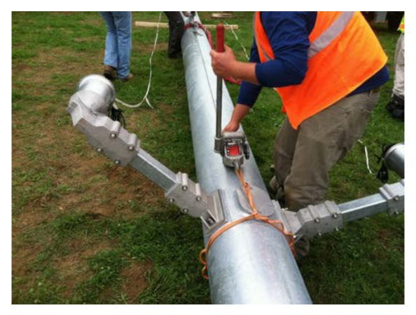
Figure 7. Multiple CLDs Attached to a Single Pole (Image courtesy of MG<sup>2</sup>)
