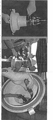
4. Using 7/16" wrench and a 7/16" Nut Driver (or 7/16" socket with extension), attach the Top –Section of the Camera Junction Box to the Bottom Contact with the included bolts/nuts/washers. (Recommended torque for 1/4" bolts is 6ft/lbs or 75 in/lbs) \*Tip: It is recommended to coat the stainless steel bolts with anti-seize lubricant prior to installing nuts
