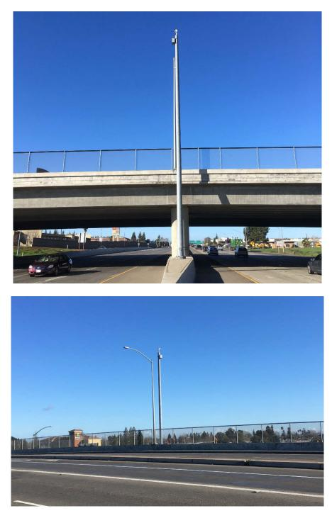
Figure 1. High-Mast Fixed Camera Mounting with Overpass Access
