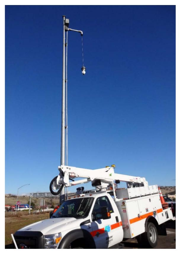
Figure 46. Lowering CCTV Camera MG2 External-Type CLD
