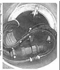
Secure Power/Signal Cable inside Pole Top Junction Box
