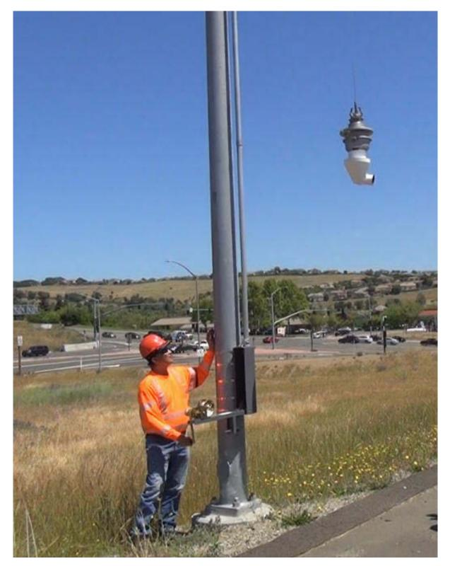
Figure 57. MG<sup>2</sup> External-Type Camera Lowering
