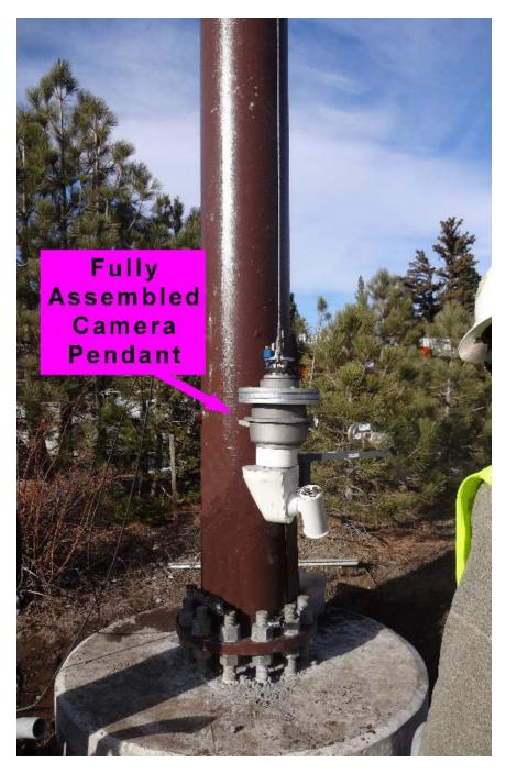
Figure 38. Fully-Assembled Camera, Pendant Lowered
