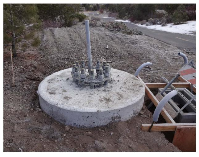
Figure 28. MG<sup>2</sup> Internal-type CLD Pole Footing
