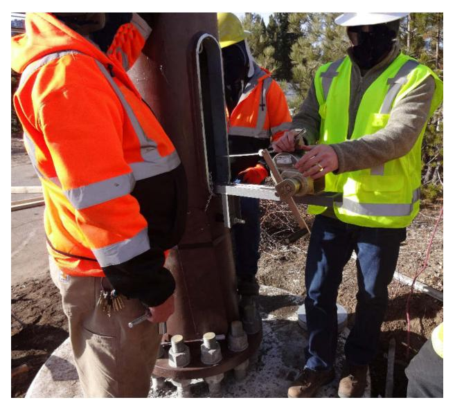
Figure 34. MG<sup>2</sup> CLD Winch Tool Attached
