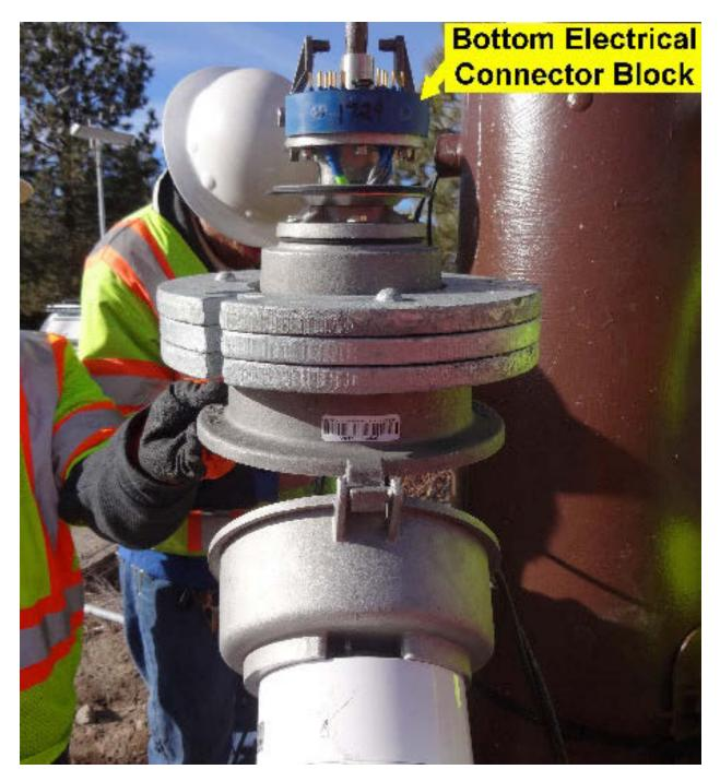
Figure 11. MG<sup>2</sup> E-Connector Installed
