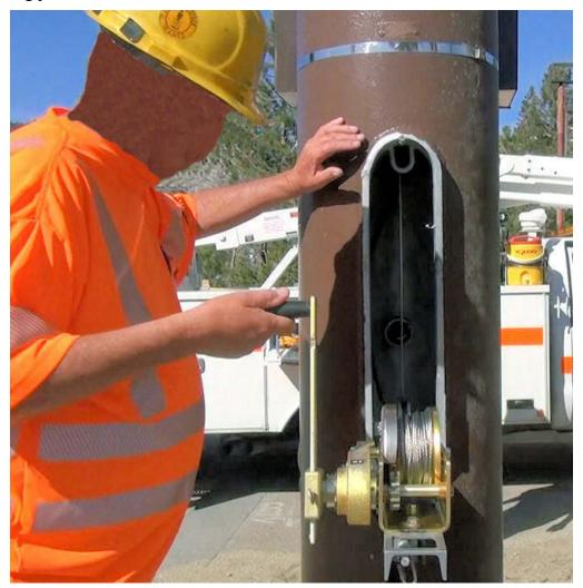
Figure 51. Hand Cranking Winch
