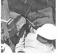
cable, engage the bottom contact and perform a continuity check Keeping slight tension on the Lowering
