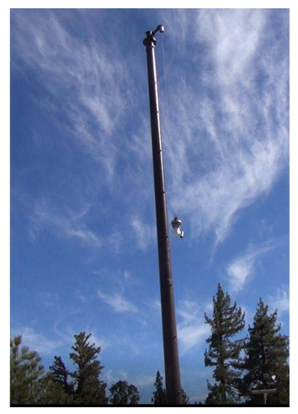
Figure 50. Meyers MG<sup>2</sup> Lowering Camera Pendant
