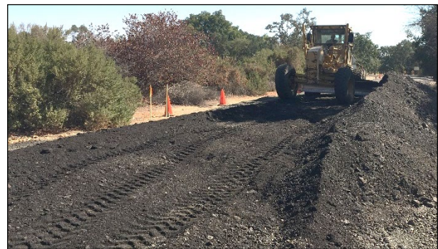
Figure 5.2: Spreading imported RAP.
