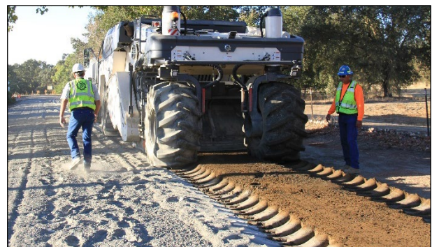
Figure 5.7: Recycled material behind the reclaimer.
