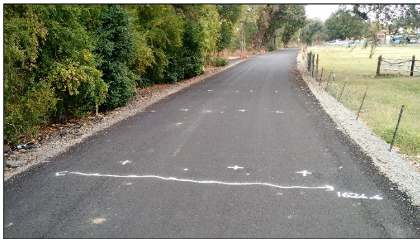
Figure 6.6: Marked crack with location.
