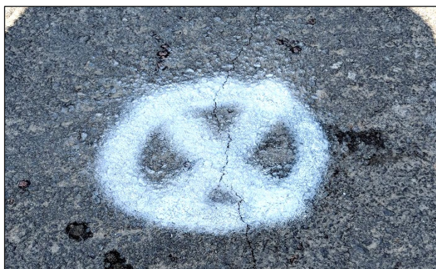
Figure 6.20: Core location through shrinkage crack.
