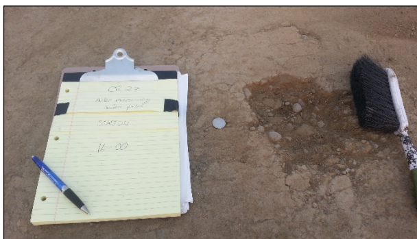
Figure 2.16: Distressed area after microcracking attributed to inappropriate curing.
