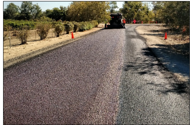
Figure 5.38: Second microsurfacing pass.
