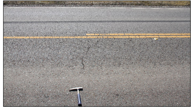
Figure 2.2: CR32B: Example transverse cracks.
