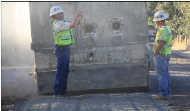
Figure 5.4: Checking cement spread rate.
