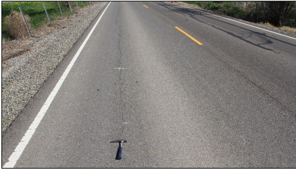
Figure 2.1: CR32B: Example longitudinal cracks.
