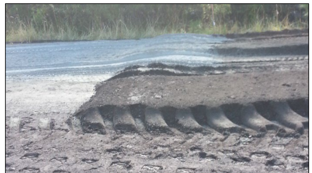
Figure 2.13: Cement spreading overlaps.
