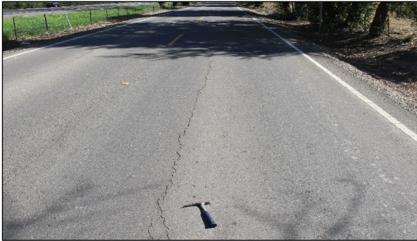
Figure 3.2: Longitudinal cracking on an FDR-C pavement.
