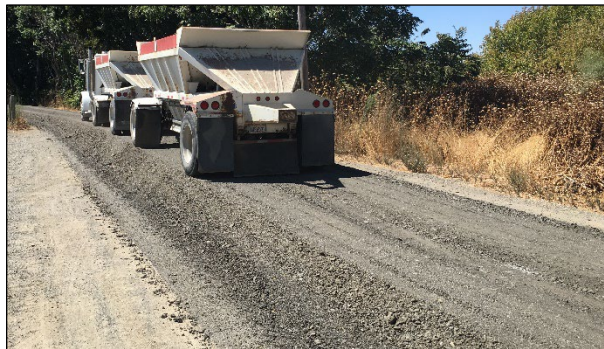
Figure 5.3: Shaped road prior to recycling.
