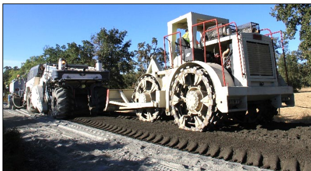
Figure 5.8: Primary compaction with a segmented padfoot roller.
