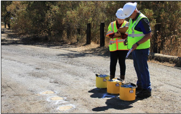
Figure 4.8: Testing with soil stiffness gauges.
