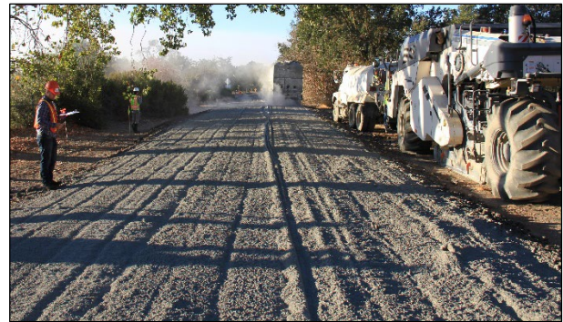
Figure 5.5: Checking cement spread overlaps.
