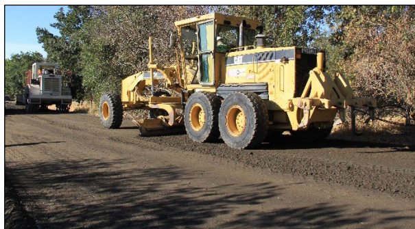
Figure 5.9: Leveling with a grader.
