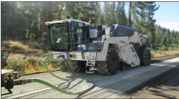
Figure 2.7: Hose dragging cement.
