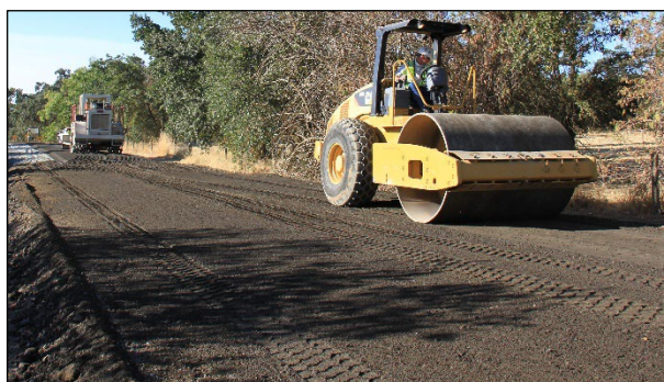
Figure 5.10: Final compaction with a smooth drum roller.
