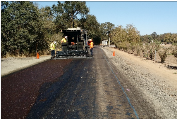
Figure 5.37: First microsurfacing pass.
