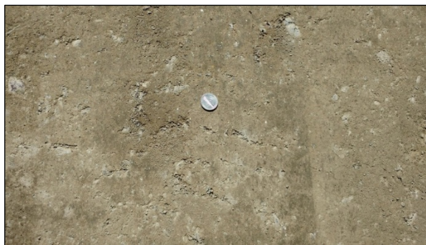
Figure 5.32: Close-up of microcracked surface.
