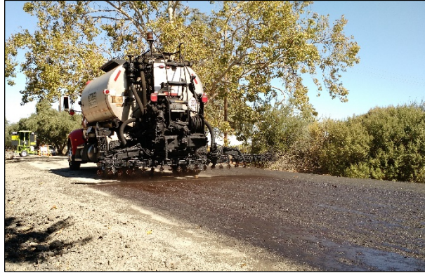
Figure 5.36: Prime coat application.
