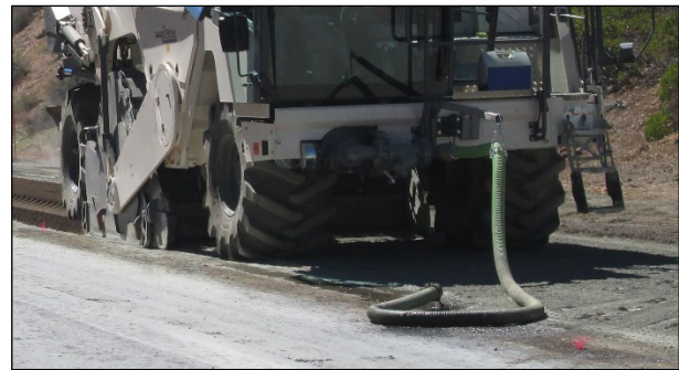
Figure 2.8: Water spill during tanker change.
