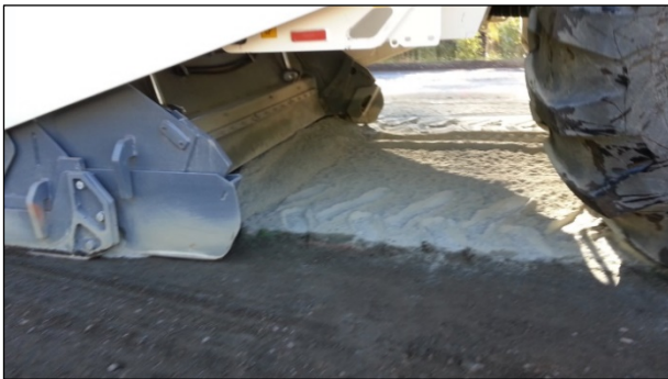
Figure 2.10: Cement redistribution in front of mixing chamber.
