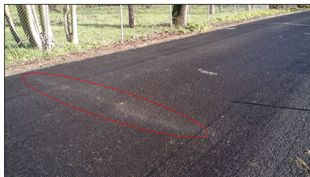
Figure 6.5: Crack identification by discoloration after water spraying.
