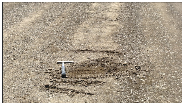
Figure 2.15: Sliver fill damaged by microcracking.
