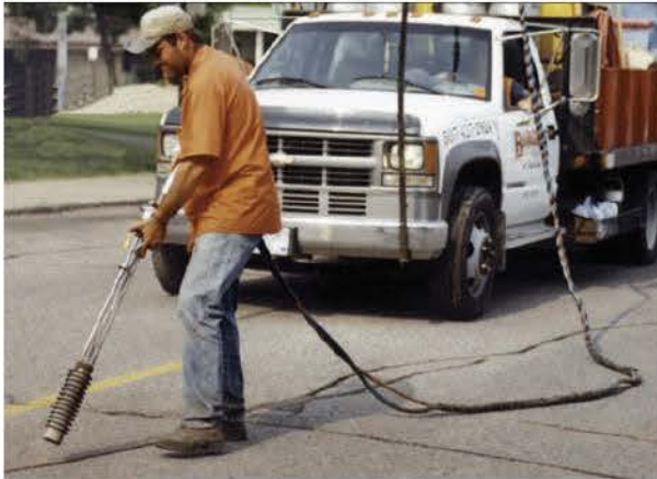
Figure 2. Heat Lance Tool (Courtesy of Cimline Mfg.)
