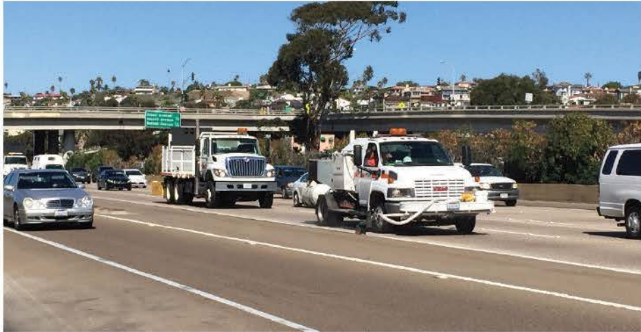
Figure 7. Vehicle-Based Sealzall Sealing in Highway Traffic on Interstate 5
