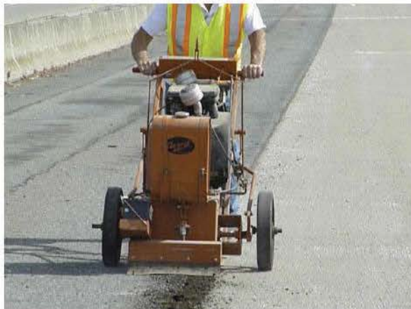
Figure 8. Standard Manual Impact Router for Joint Crack Cleaning
