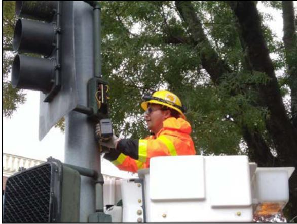
(c) Drilling hole in the small wire box on the signal pole
