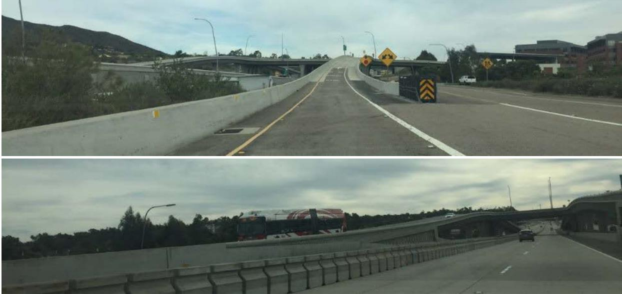
**Fig 20. Direct Access Ramps on I-15 for Public Transit.**
