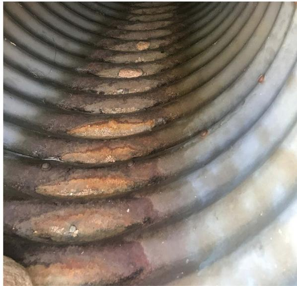
**Fig. 3.6** Moderate corrosion from agricultural land due to acidic soil and high bacteria content
