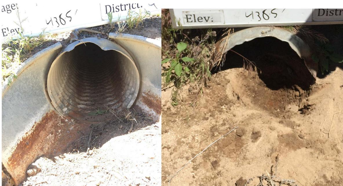
**Fig. 3.1** Left: light corrosion, Right: completely corroded
