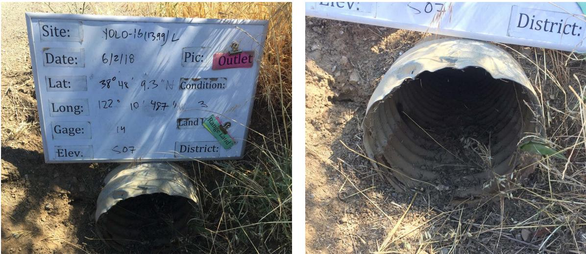
**Fig. 3.4** Left: a culvert with a score of 3, Right: a closer look at the invert
