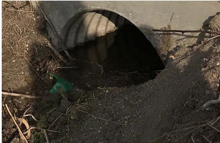
**Fig. 3.2** Low slope accumulates standing water due soil at culvert outlet
