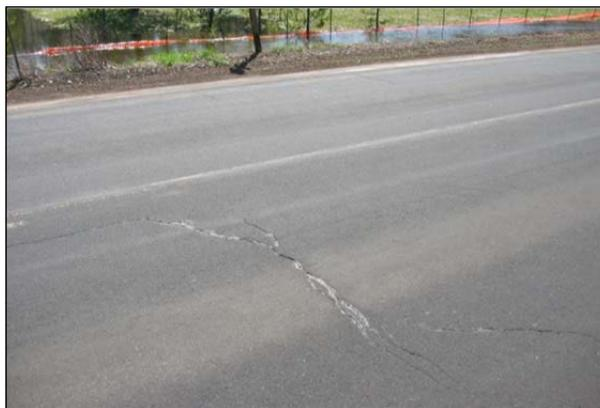
**Figure 2.1: Transverse crack.**
