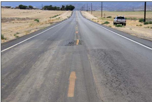
**Figure 2.5: Fatigue cracking.**
