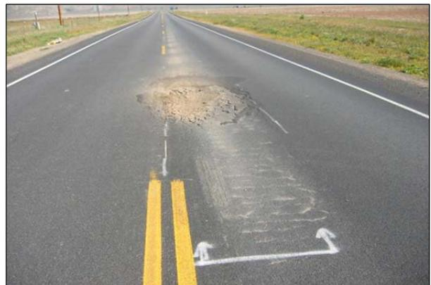
**Figure 2.6: Pumping through fatigue cracking.**
