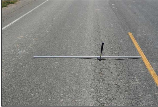
**Figure 2.7: Rutting caused by water ingress through cracks into the base.**
