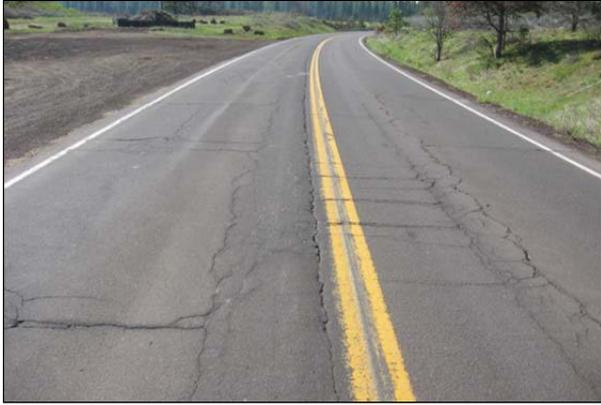
**Figure 2.3: Block cracking.**
