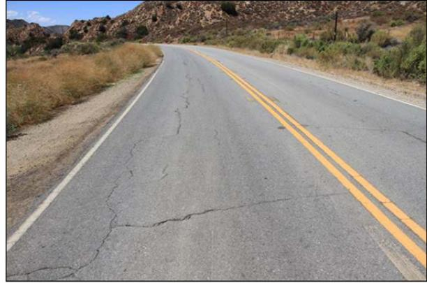
**Figure 2.4: Block crack progression.**
