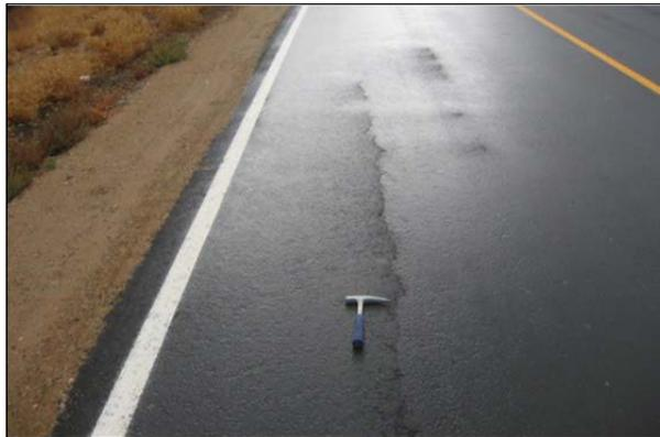
**Figure 2.2: Longitudinal crack.**
