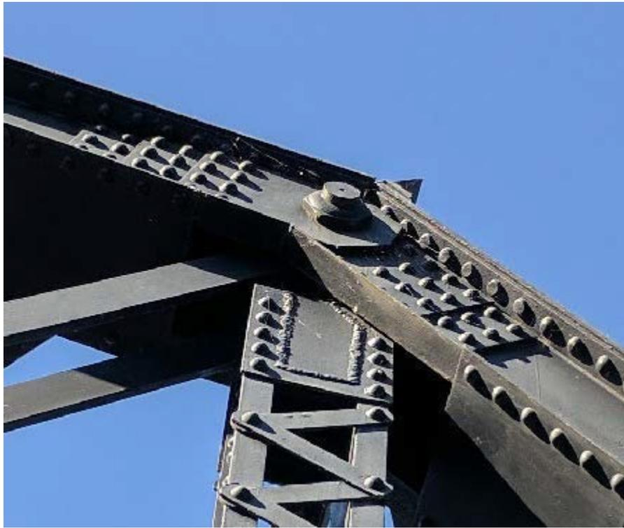
Figure 2-2: Pin plates at pinned truss joints.
