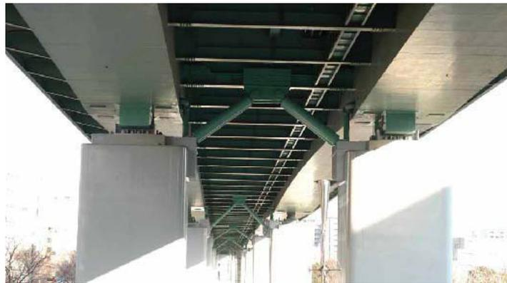
**Figure 2.8 BRBs Used as Ductile Diaphragm (Japan)**
