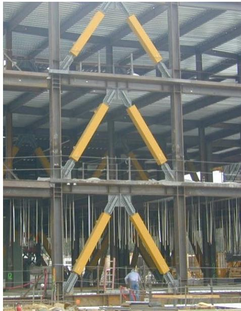
Figure 2.2 Typical BRB Frames within a Building Structure
