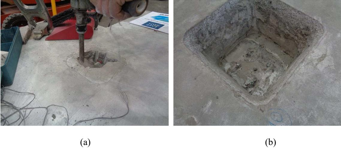
**Figure 2-35 Grout Removal**
