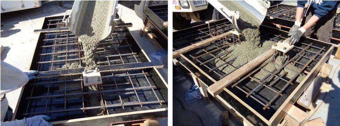
**Figure 2-10 Concrete Pouring on Girder Specimens**
