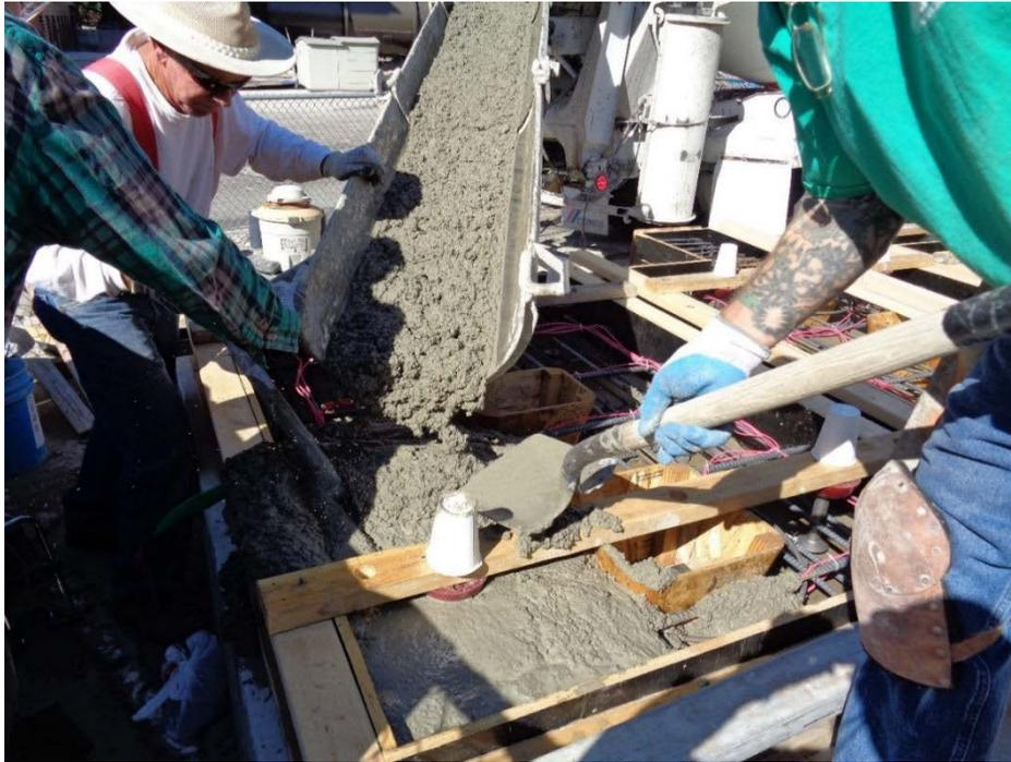
**Figure 2-4 Concrete Pouring on Deck Specimens**
