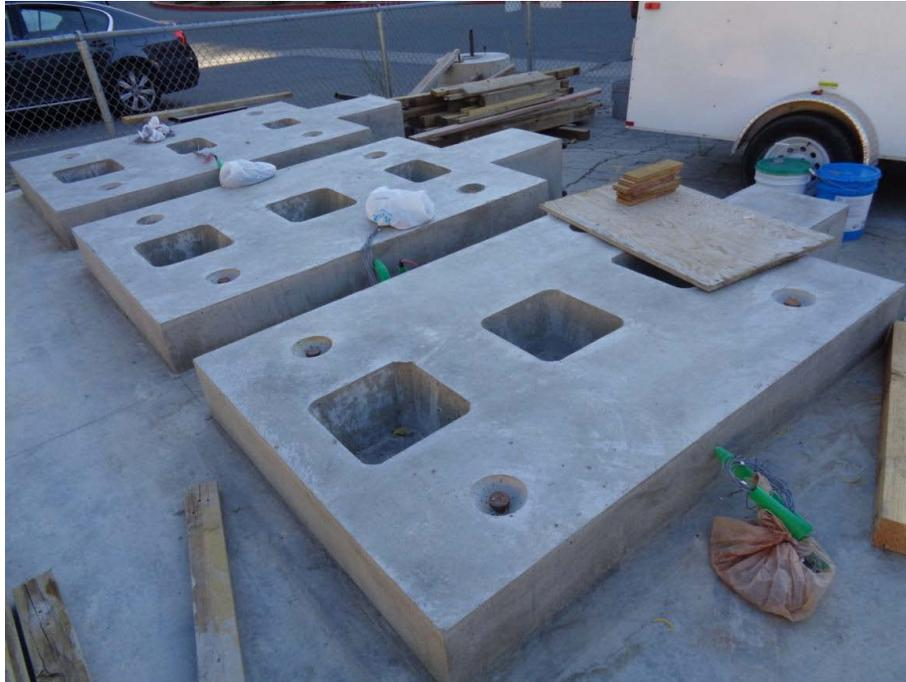
**Figure 2-6 Deck Sections with Voided Pockets**
