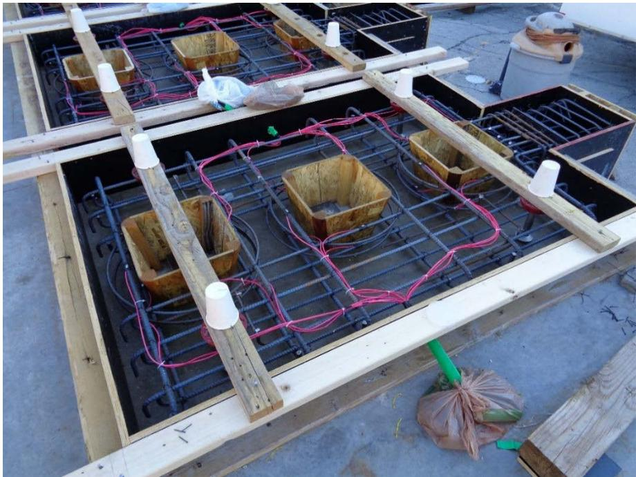
**Figure 2-3 Deck Reinforcement Details**
