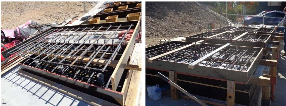
**Figure 2-9 Girder and Footing Reinforcement Details**
