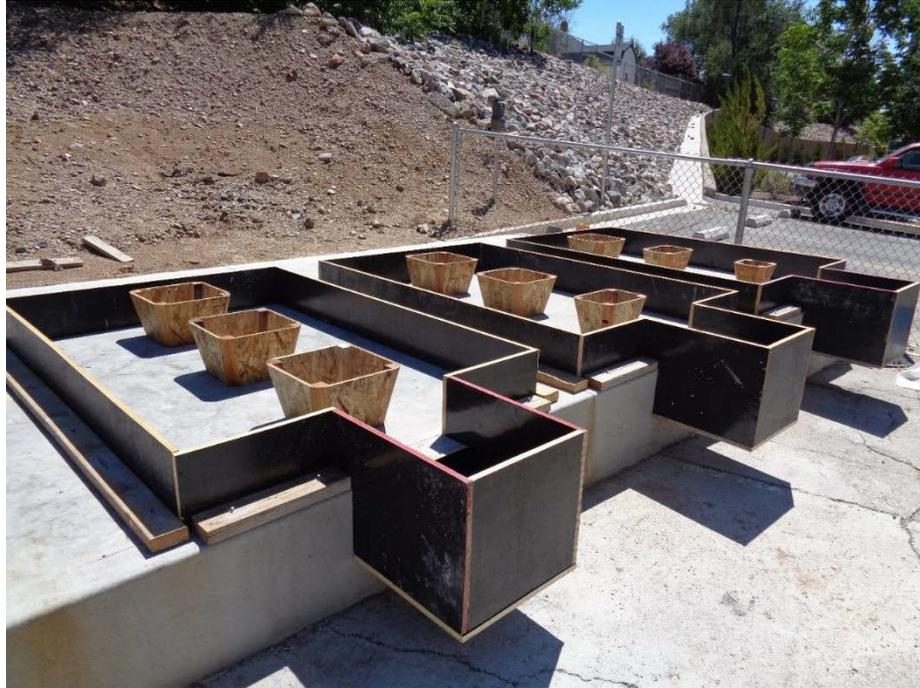
**Figure 2-2 Formwork for Deck Specimens with Grout Pockets**
