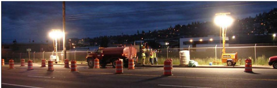
**Figure 3. Balloon Lighting at a Highway Work Zone.**
