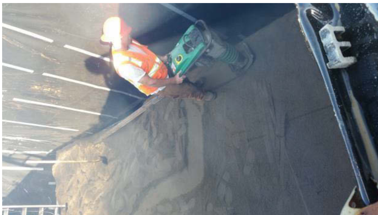
Figure A-8: Backfill compaction
