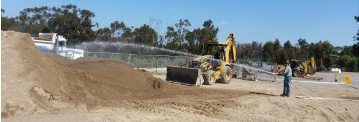
Figure A-5: Adjusting soil moisture
