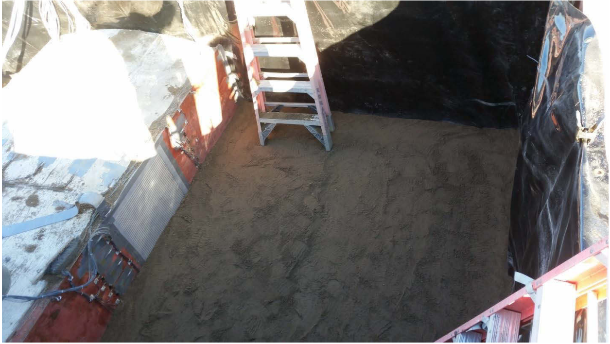
Figure A-12: Backfilling
