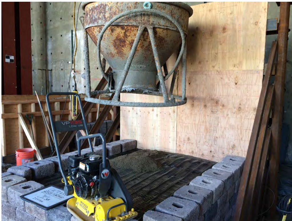
Figure A2.8 Concrete hopper to dump sand.
